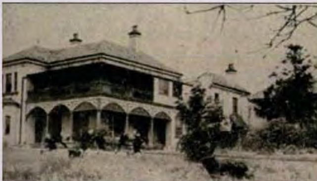
4. View of southern side of the Orphanage. Note what appears to be a Norfolk Island Pine in the right of the photograph. (Source: http://uonccmayfield.files.wordpress.com ).
