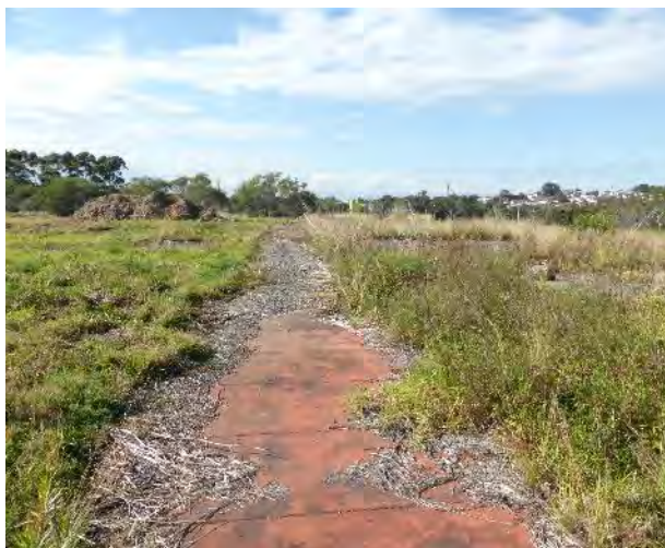
Figure 7 Remains of the orphanage concrete path
