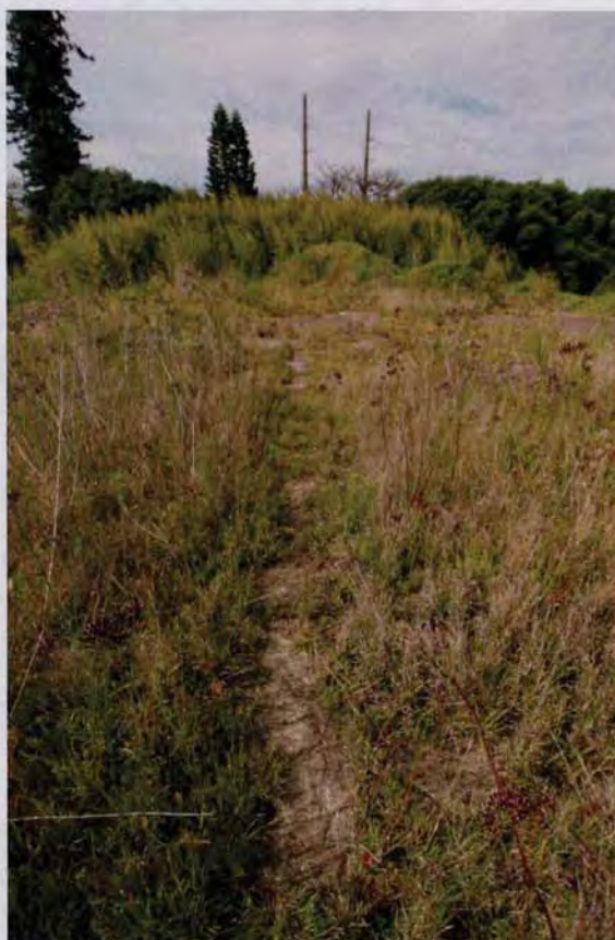
Figure 6 View looking north, showing (overgrown) sandstone footing, and Cook Island pine plus seedlings in background. source: Heritas December 2013
