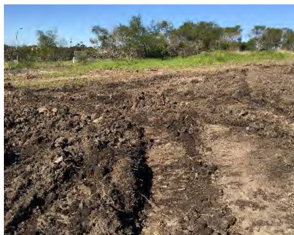
Figure 25 Clean topsoil after removal of vegetation
