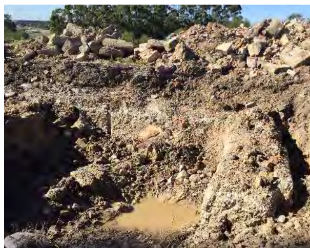
Figure 19 Concrete and brick foundations and remains of the cellar of the Superintendent's house
