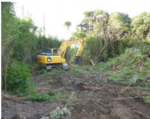
Figure 20 Removal of vegetation (bamboo) in the northern part of the site
