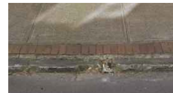
Standard brick pavers and concrete (Bishopsgate Street, Wickham)
