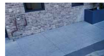
Pavement type 3 (PT3) stone and concrete with just one line of bluestone pavers
