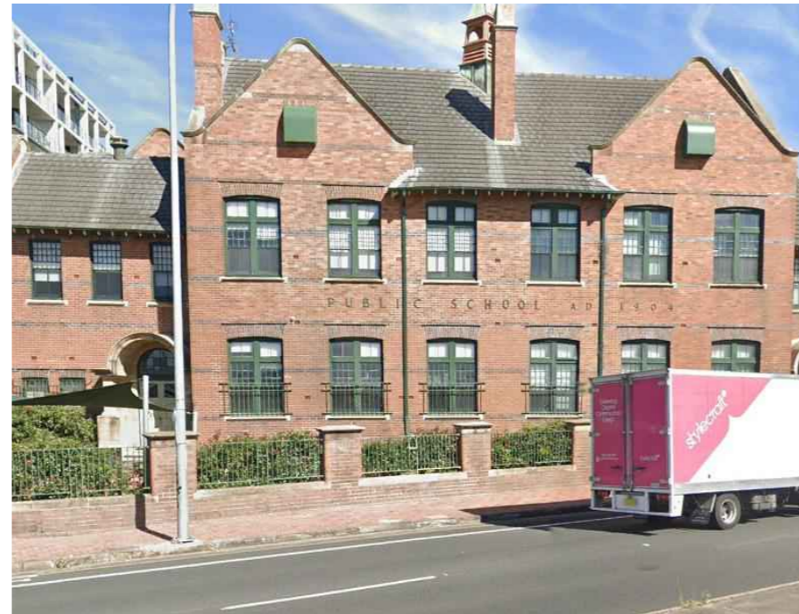
Former Wickham Public School, Hannell Street
