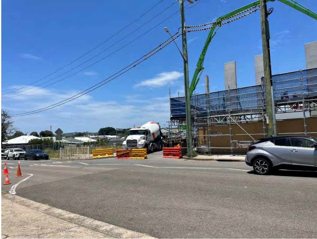
Looking towards Turner Street and construction occurring
