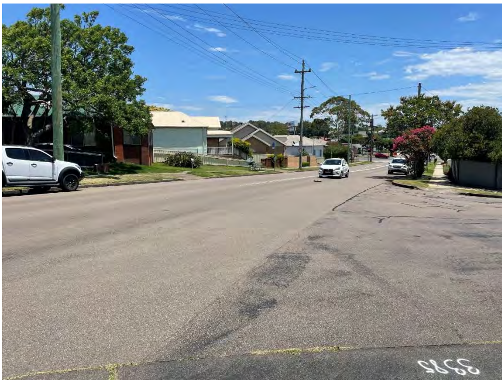
Georgetown Road / Bowker Street intersection.
