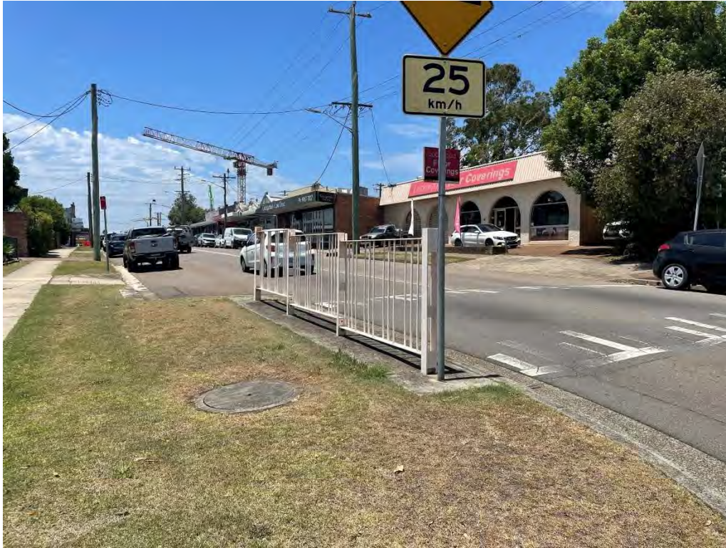
Existing threshold looking east along Georgetown Road
