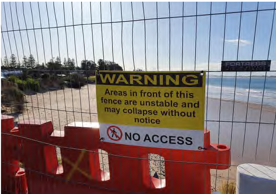
Figure 26: Facing north showing no access from the northern breakwater.
