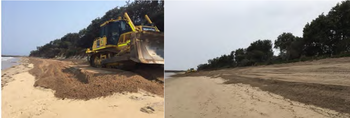
Figure 9: Photographs from the December 2019 pilot nourishment campaign (left) in progress and (right) upon completion (source: RHDHV, 2020).
