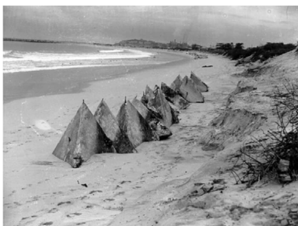
Figure 31: Anti-tank traps along Stockton Beach in the 1940s. Source: Newcastle Regional Library.
