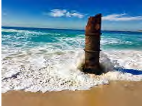
Figure 46: Potential Stockton Colliery ventilation pipe which has since washed away. 92
