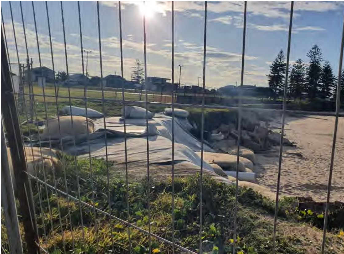
Figure 27: Facing north showing coastal protection works adjoining public recreation spaces.
