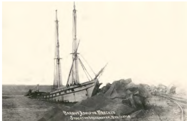
Figure 22: The Adolphe incorporated into the Stockton Breakwater. Date Unknown. 60
