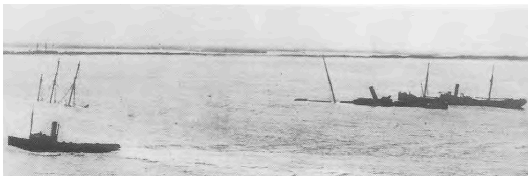
Figure 23: Stockton Breakwater wrecks, from left to right, Regent Murray, Wendouree and Lindus. Passing tug in the foreground. Date Unknown. 61
