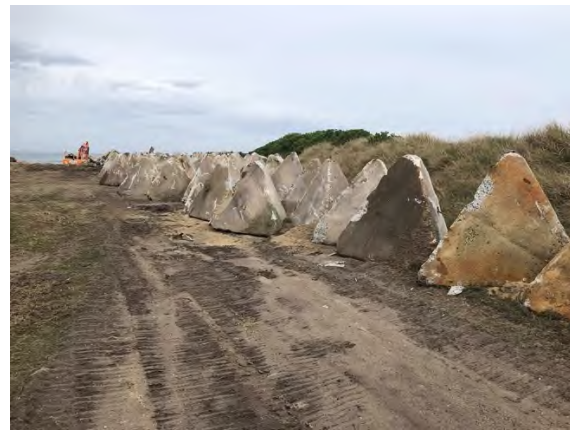
Figure 34: Concrete tank traps removed by Hunter Water. Image: Hunter Water.
