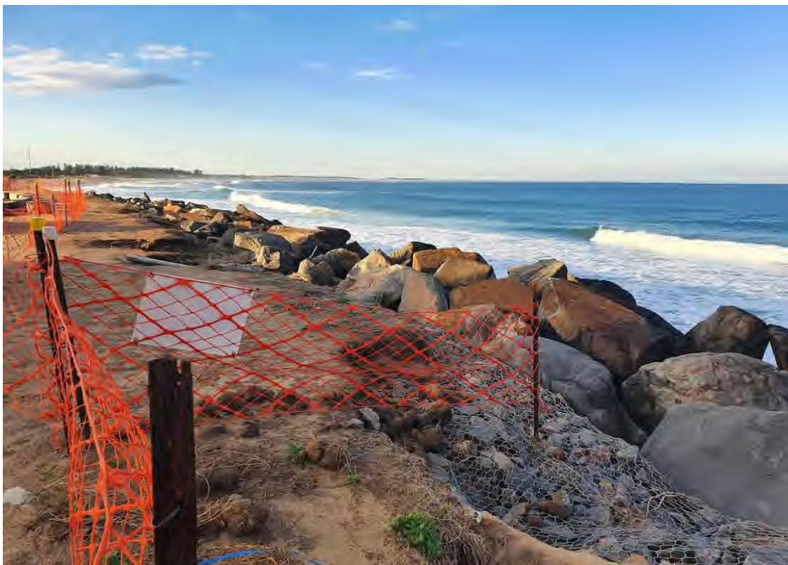
Figure 28: Facing north showing gabion baskets and rock protection.
