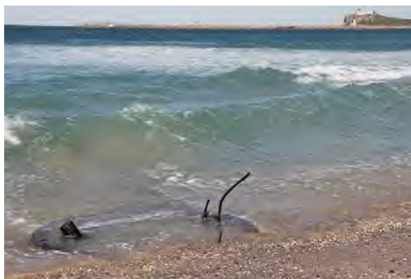
Figure 30: Stockton No. 3 Shaft exposed at 0.35m low tide in September 2017. The shaft has a diameter of approximately 3m. Remains of ladder can be seen on right. Photographer: Russell Rigby. Source: Hunter Living Histories.
