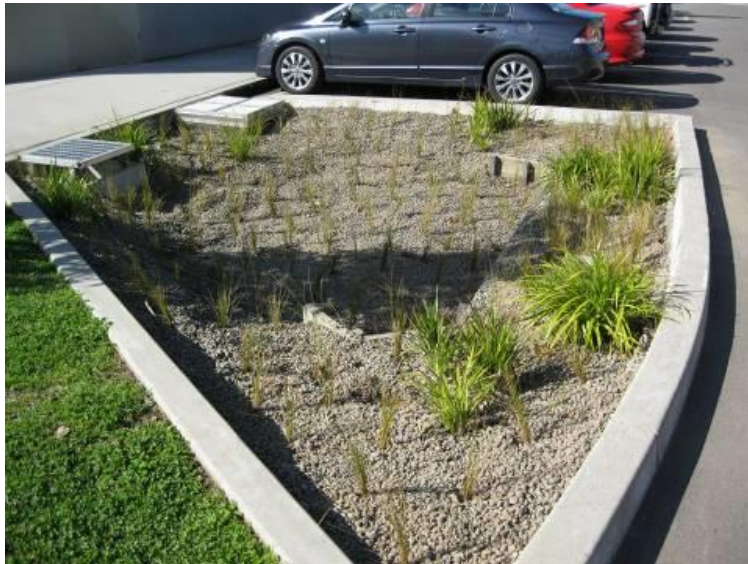
Figure 4.6.1 - Bioretention rain garden
