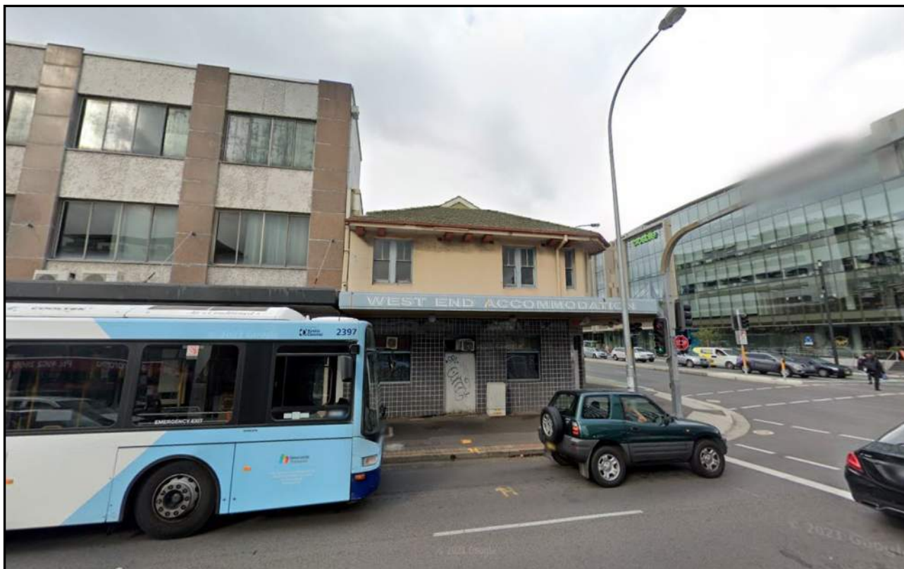
Photo 3: View of subject site looking south from Hunter Street, (Google Maps, 2022).
