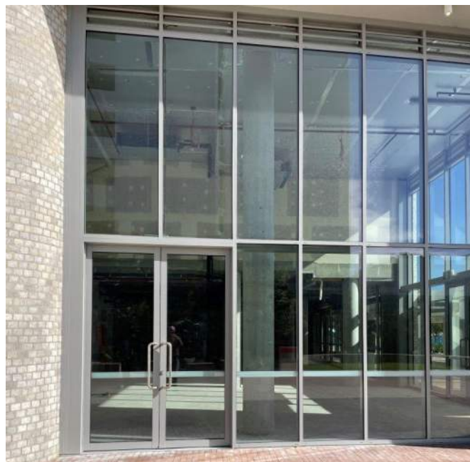
Figure 4. View from east of ground floor glazing.
