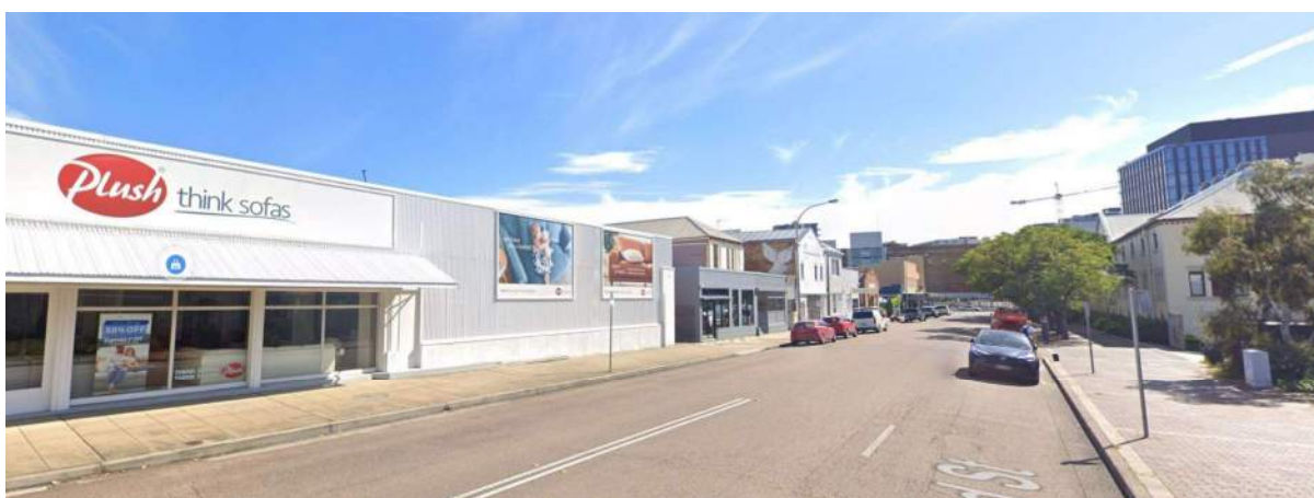
Figure 130: 22 Wood Street, Newcastle West facing north (Source: Google Streetview)
