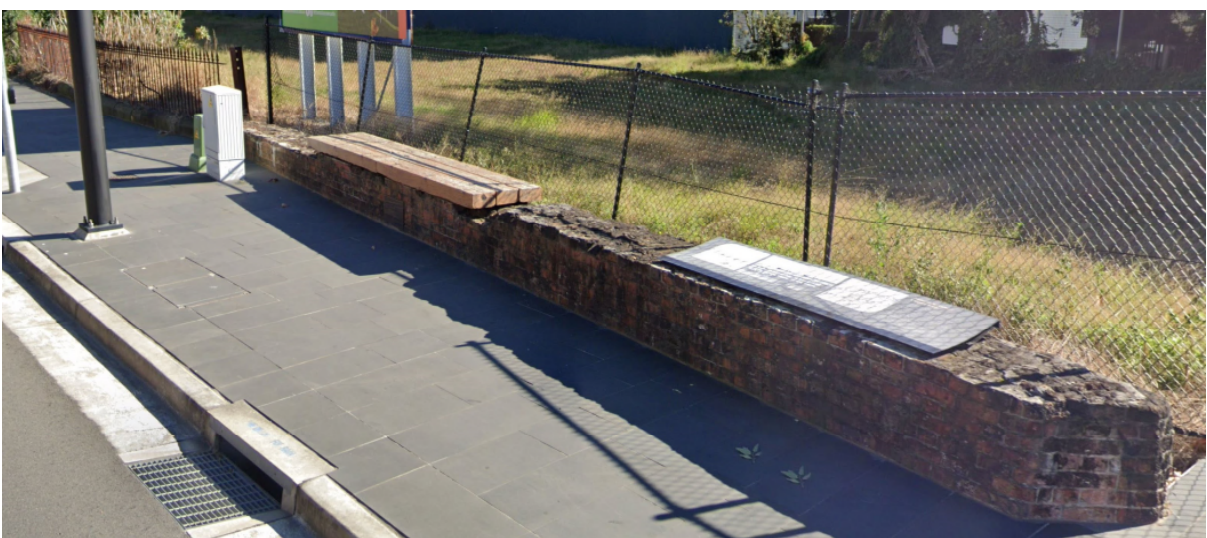
Figure 88: remains of AA Company Bridge and Fence at 280 Hunter Street (Source: Google Streetview)
