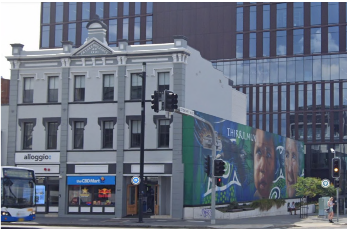
Figure 136: 840 Hunter Street, Newcastle West (Source: Google Streetview)
