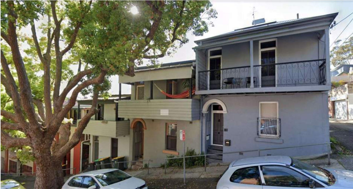
Figure 67: 15, 17 and 19 Brown Street, Newcastle (Source: Google Streetview)
