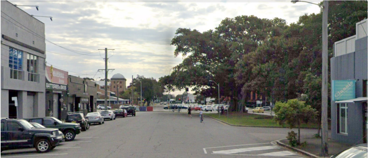
Figure 120: 69 and 154 Parry Street, Newcastle West - view north towards Stewart Avenue (Source: Google Streetview)
