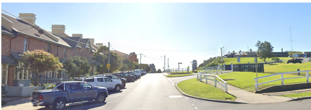
Figure 34: Boatman's Terrace Group and Fort Scratchley, Newcastle East facing north (Source: Google Streetview)
