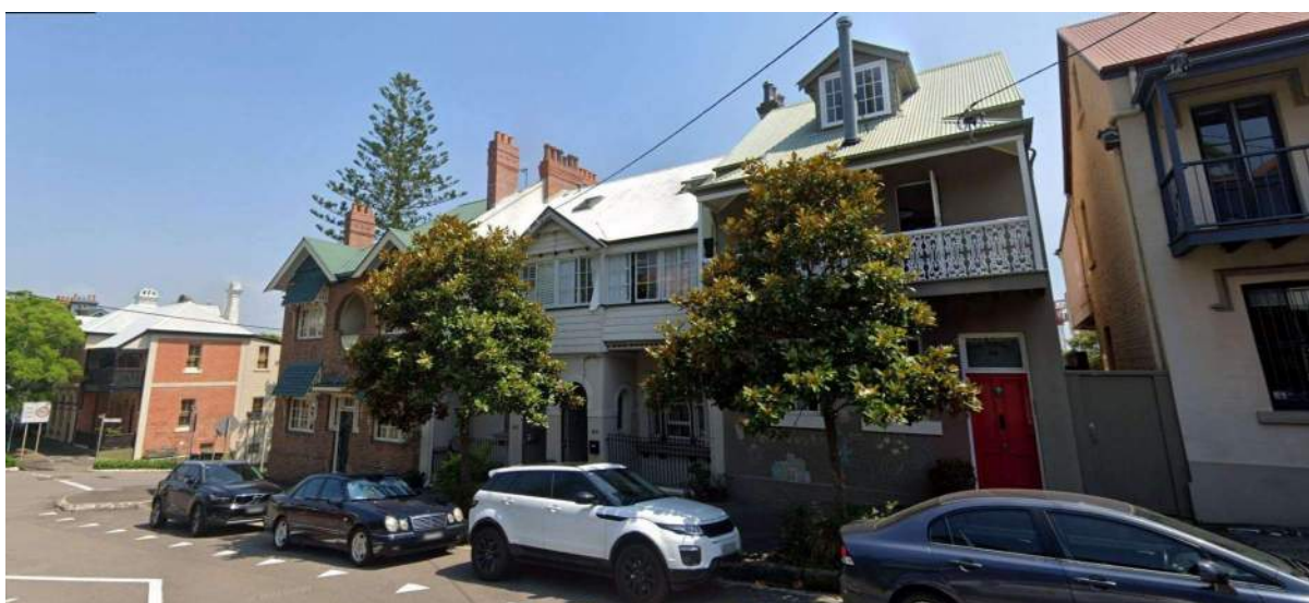
Figure 65: 58 Church Street, The Hill facing west (Source: Google Streetview)
