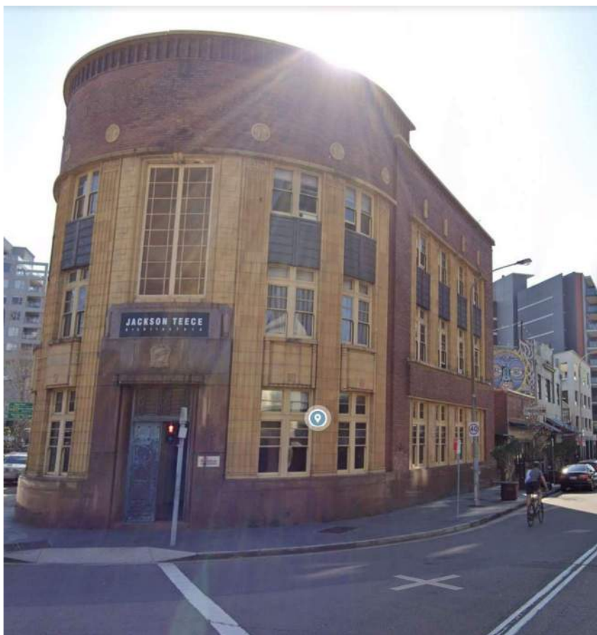
Figure 105: Bank Corner at 744 Hunter Street, Newcastle West (Source: Google Streetview)
