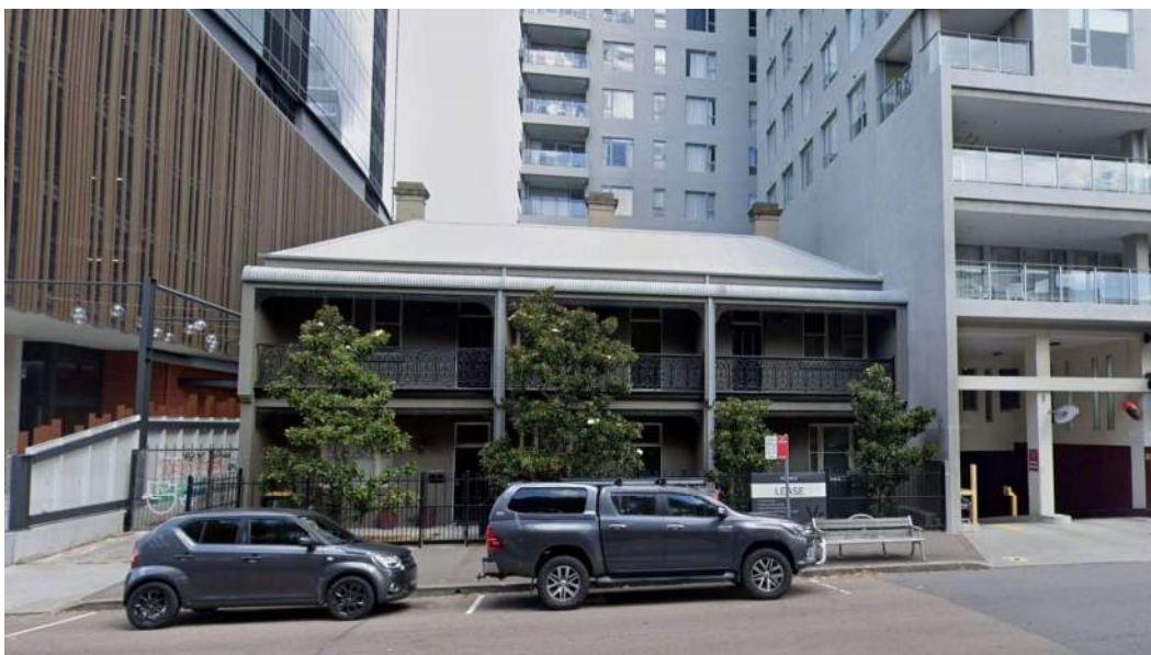
Figure 134: 741 Hunter Street, Newcastle West (Source: Google Streetview)
