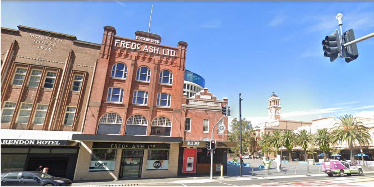
Figure 75: Wheeler Place facing south (Source: Google Streetview)
