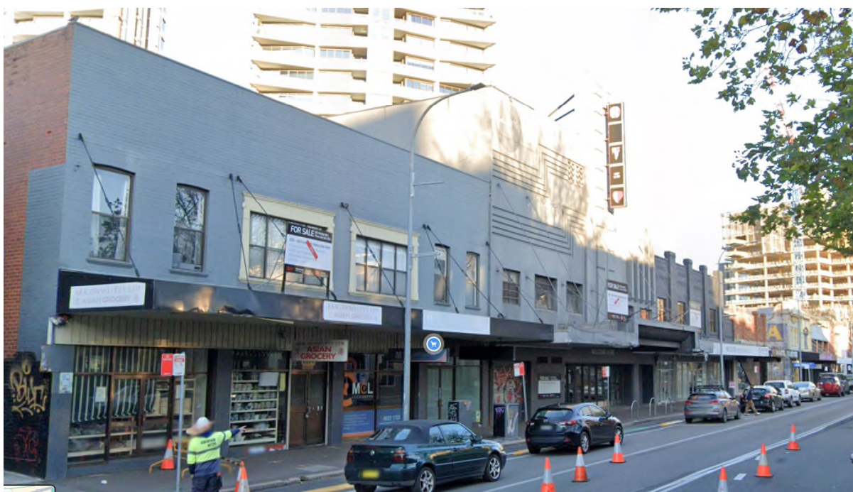
Figure 104: Theatre Royale at 669 Hunter Street, Newcastle West and its neighbours (Source: Google Streetview)
