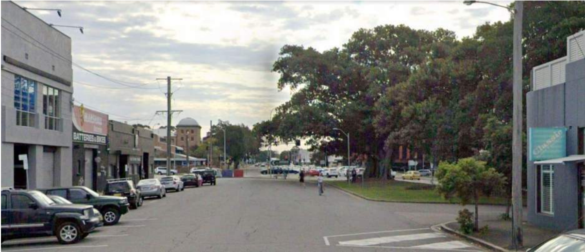
Figure 120: 69 and 154 Parry Street, Newcastle West - view north towards Stewart Avenue (Source: Google Streetview)
