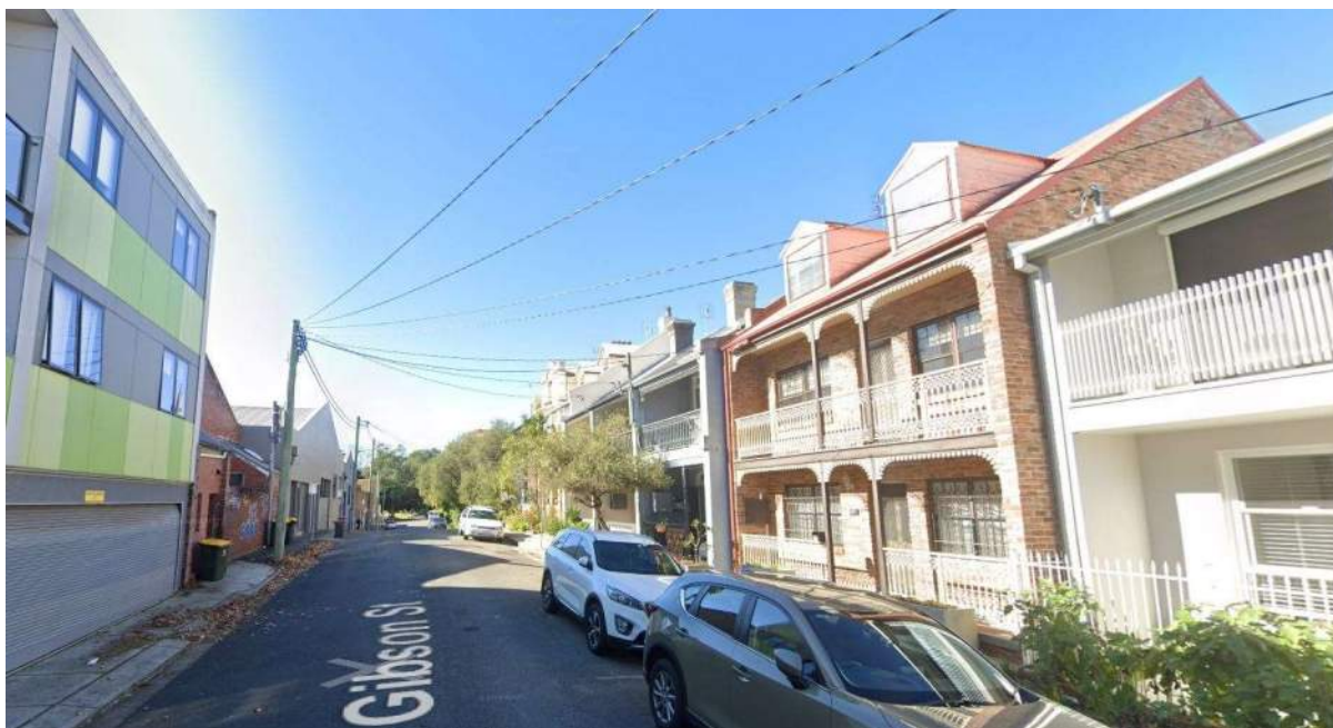
Figure 92: 43 Gibson Street and rear of 267 King Street, Newcastle facing east (Source: Google Streetview)
