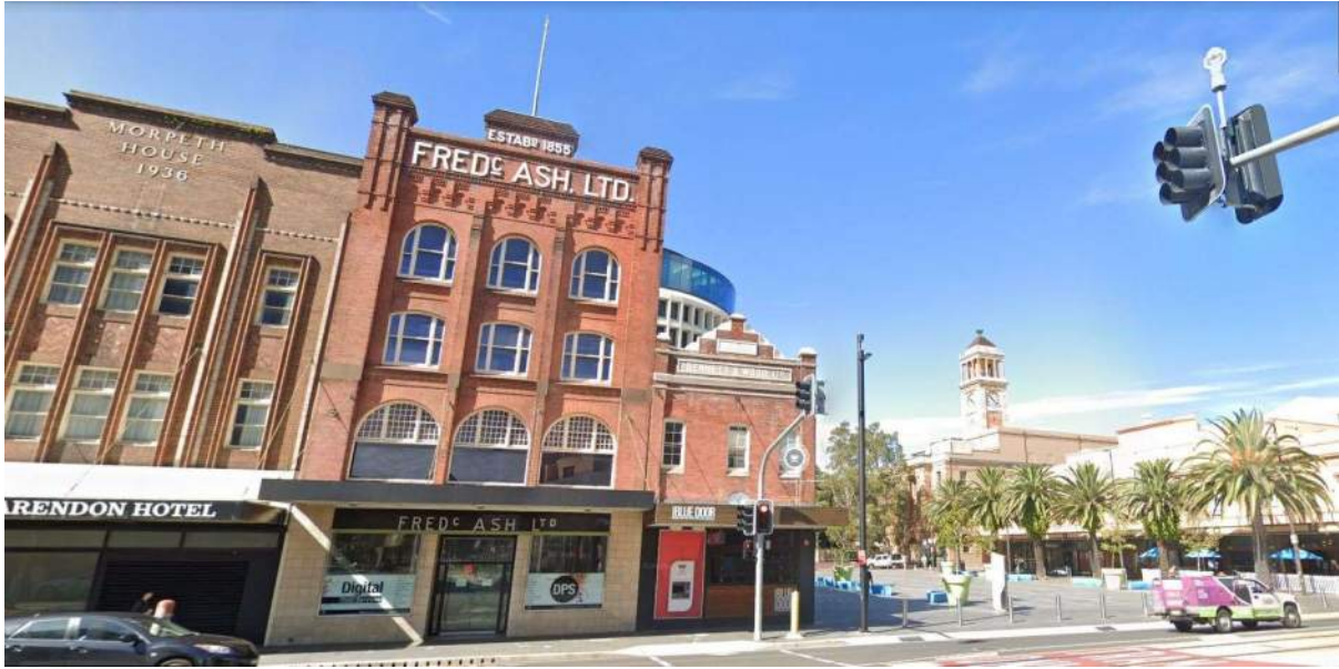
Figure 75: Wheeler Place facing south (Source: Google Streetview)
