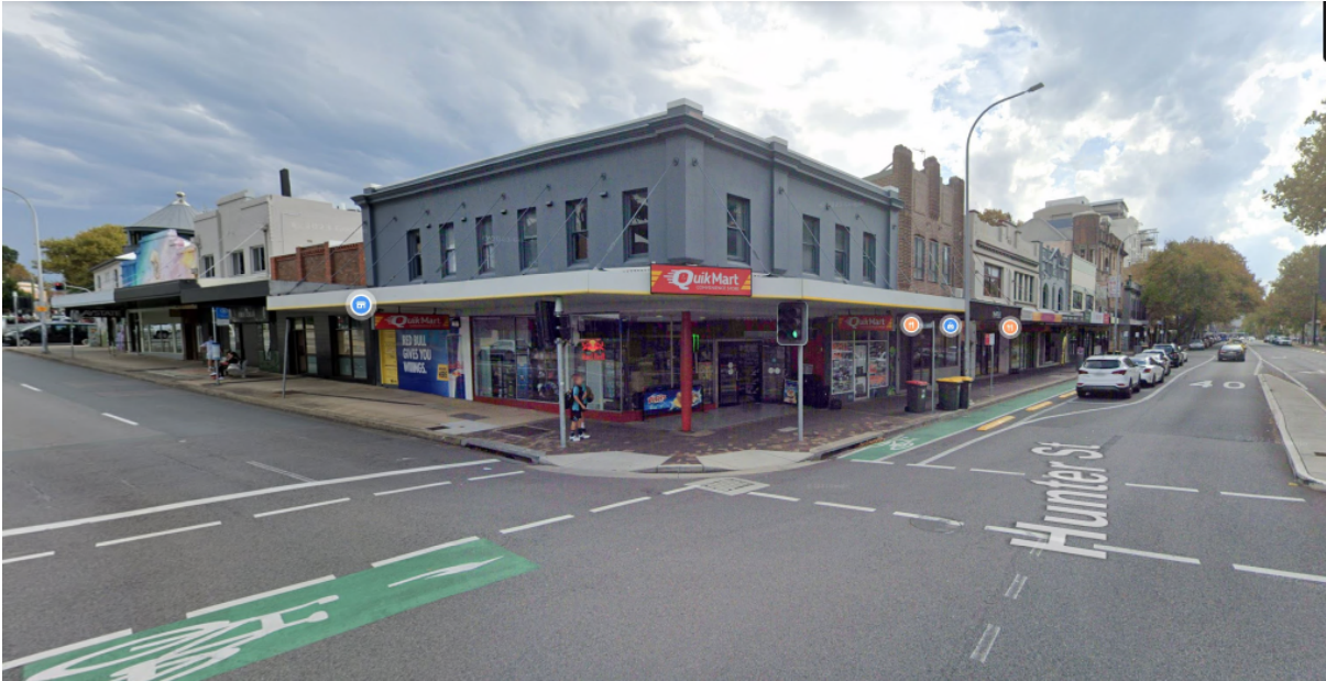
Figure 99: Corner of Union and Hunter streets, Newcastle West facing west (Source: Google Streetview)
