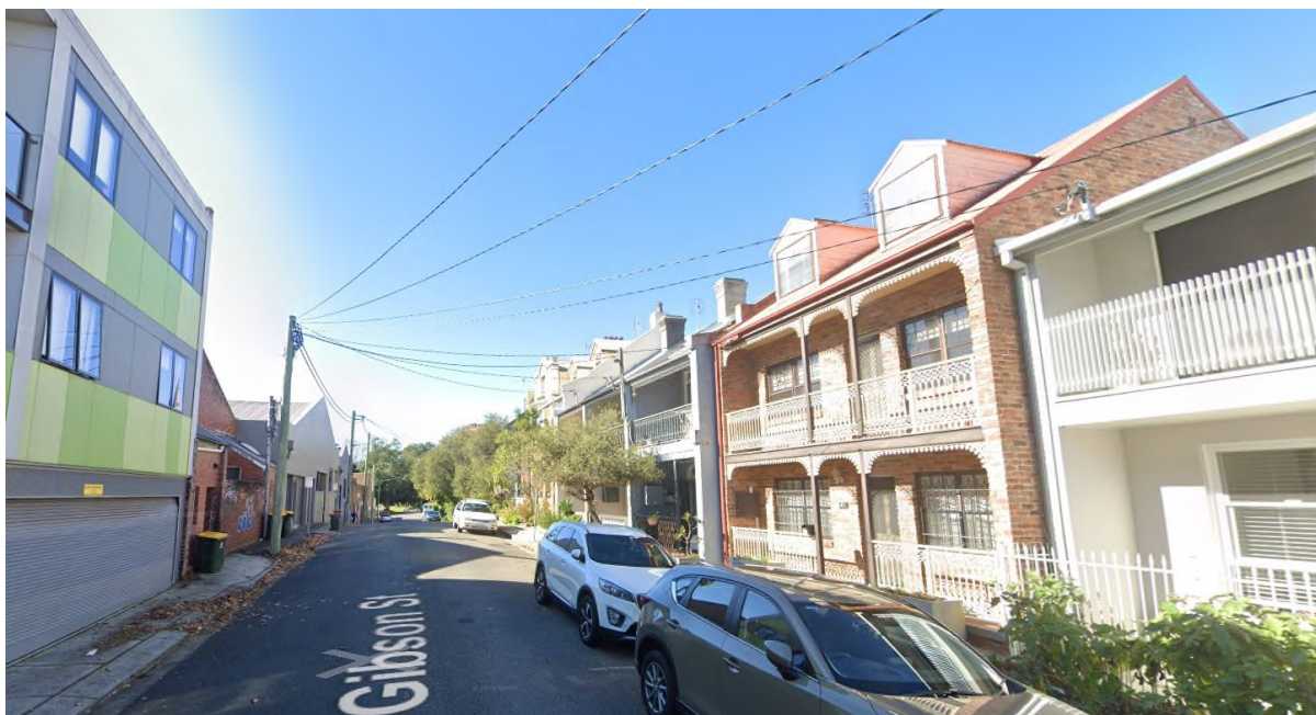
Figure 92: 43 Gibson Street and rear of 267 King Street, Newcastle facing east (Source: Google Streetview)
