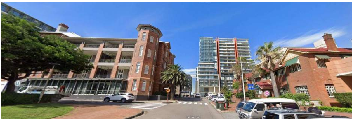
Figure 56: Newcastle Hospital North Wing at 2 Ocean Street and Former Nurses' Home (Royal Newcastle Hospital - The Club Building) at 30 Pacific Street, Newcastle (Source: Google Streetview)
