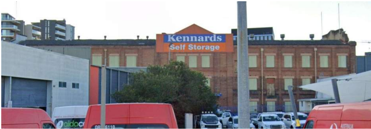
Figure 137: 904-908 Hunter Street, Newcastle West (Source: Google Streetview)
