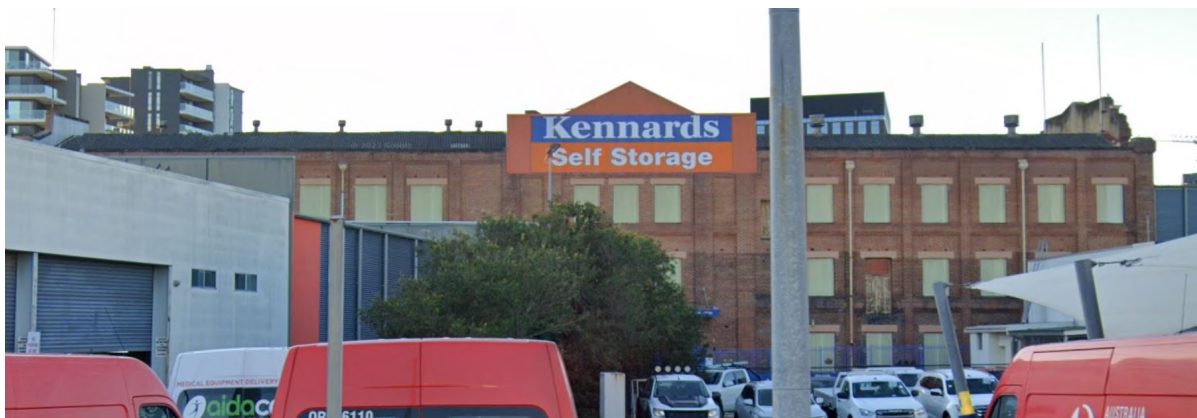
Figure 137: 904-908 Hunter Street, Newcastle West (Source: Google Streetview)
