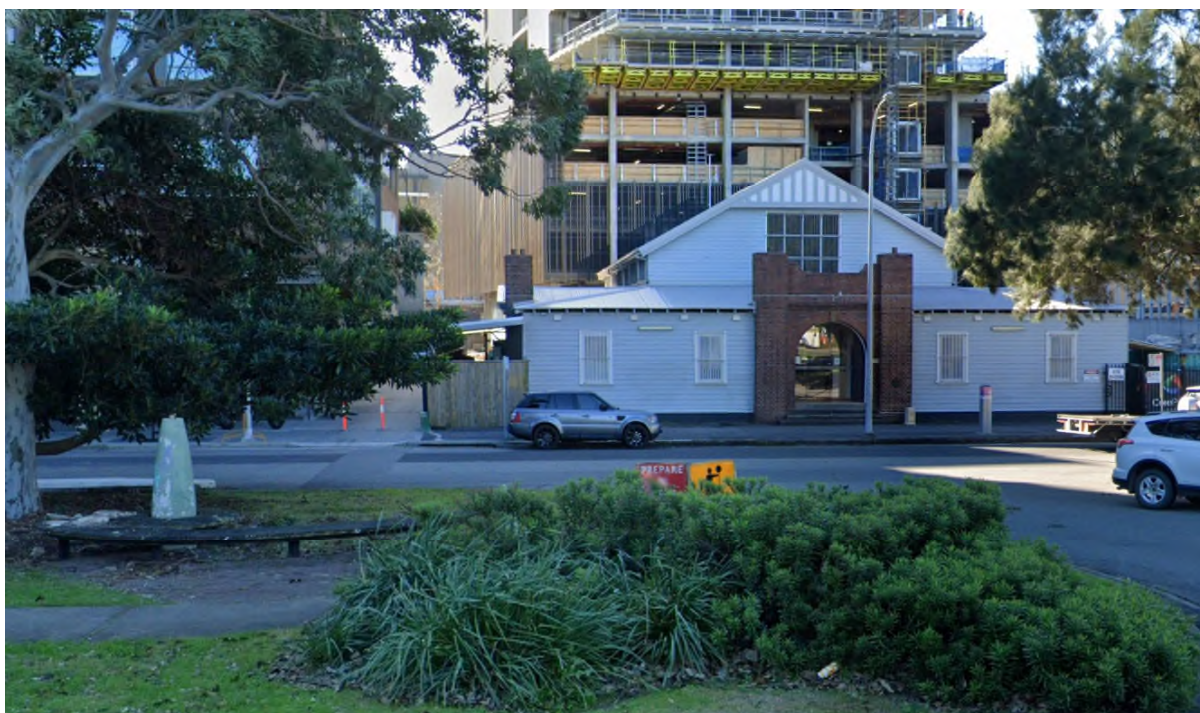
Figure 132: Birdwood Park and the Army Drill Hall at 498 King Street, Newcastle West (Source: Google Streetview)
