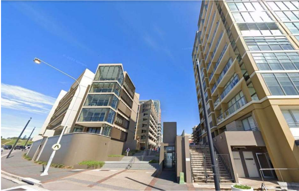
Figure 61: 61 Shortland Esplanade and 1 King Street, Newcastle (Source: Google Streetview)
