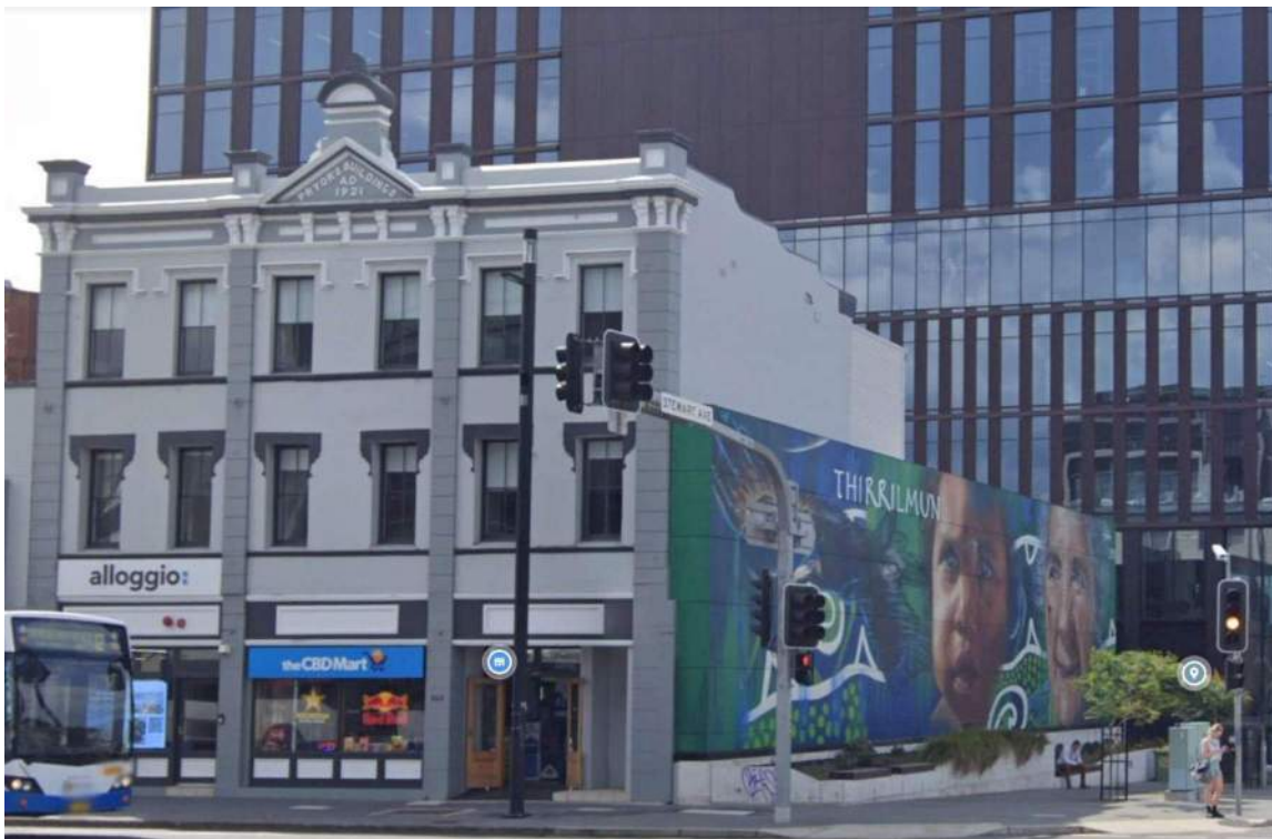
Figure 136: 840 Hunter Street, Newcastle West (Source: Google Streetview)
