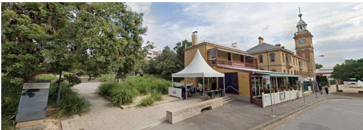
Figure 29: Convict Lumber Yard, Paymasters Cottage, and Newcastle Customs House, Newcastle East (Source: Google Streetview)
