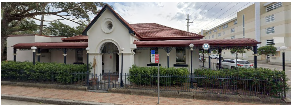
Figure 85: Fanny's Tavern at 311 Wharf Road, Newcastle (Source: Google Streetview)
