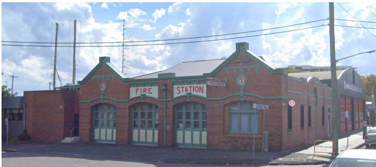
Figure 113: Fire Station at 44 Union Street, Cooks Hill (Source: Google Streetview)
