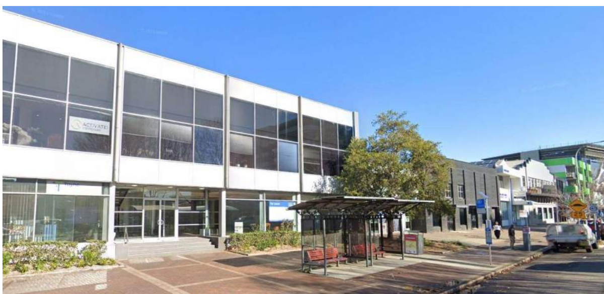
Figure 91: 239 King Street, Newcastle facing west (Source: Google Streetview)
