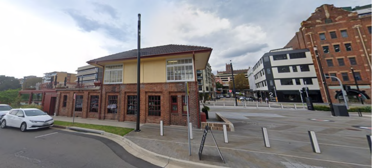
Figure 54: Newcastle Signal Box at 155 Wharf Road, Newcastle with the tower of Christ Church Cathedral in background (Source: Google Streetview)
