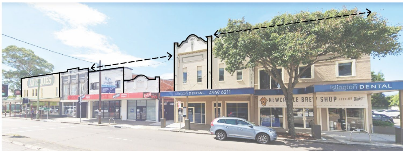
Figure 37: Existing parapets dominating the street edge
