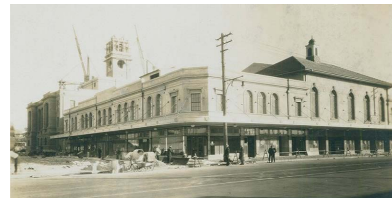
Builders put the finishing touches on Civic Theatre as work progressed on City Hall's clocktower.
