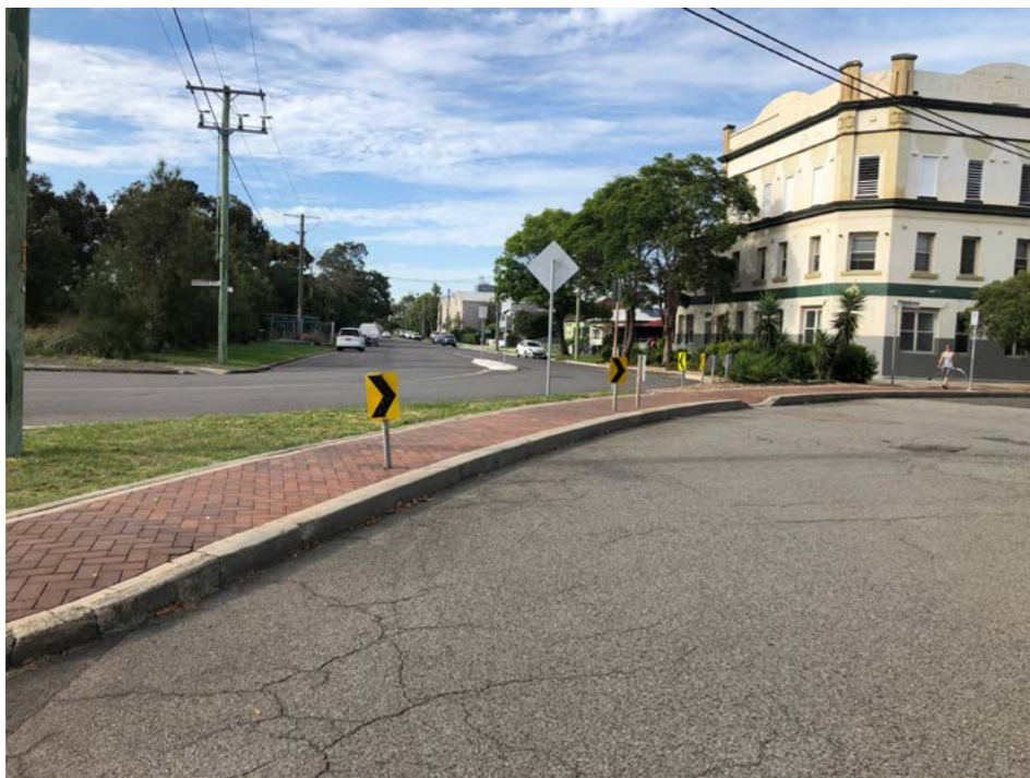
Figure 19 Existing Road block Bourke/Robertson Streets
