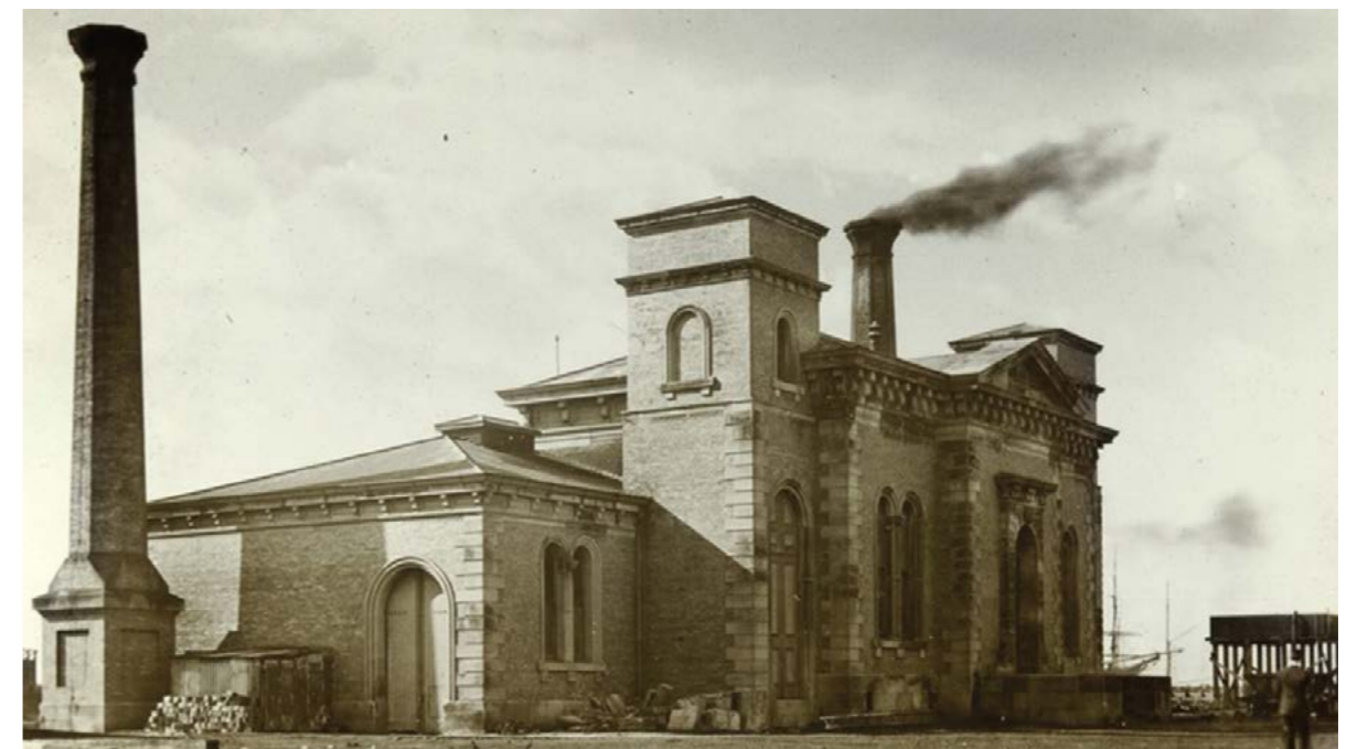
Figure 16 State heritage listed Carrington Pump House which was NSW's first large scale hydraulic power system (Source: State Library of Victoria)
