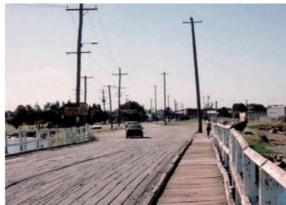
Figure 6 Cowper Street Bridge pre reconstruction on in 1992. (Source: Hunter and Central Coast Development Corporation)
