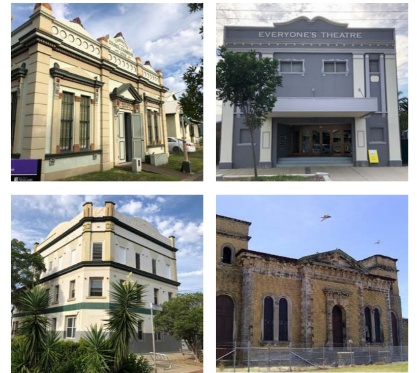
Figure 15 Selection of Heritage listed buildings in Carrington including the Council Chambers (top left), Everyone's Theatre (top right), Carrington Club Hotel (bottom left) and the Carrington Pump House (bottom right)
