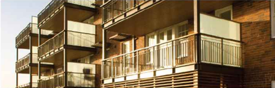
Timber coastal apartments - Wood Solutions
