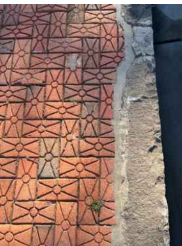
Figure E2.34: Heritage road assets such as sandstone kerbing and restored historic pavements.
