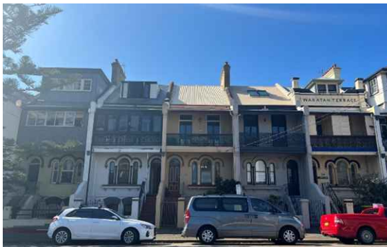
Figure E2.28: Row of three-storey terraces demonstrating the regular pattern of subdivision, ornate elements present in buildings constructed from mid-19 th and early 20 th centuries.
