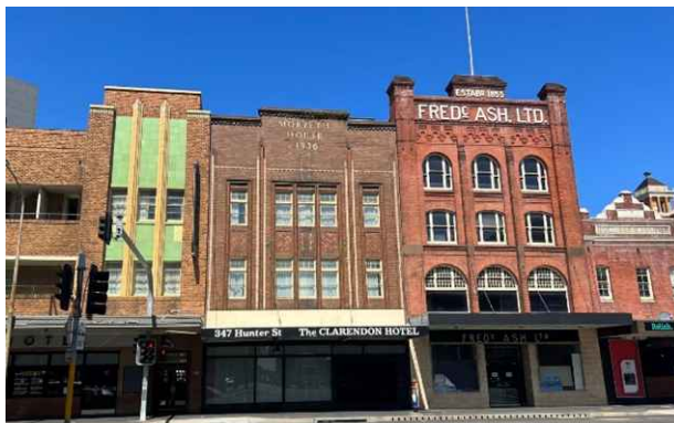
Figure E2.24: Buildings built in mid-19 th to early 20 th centuries enhance the rich historic character.
