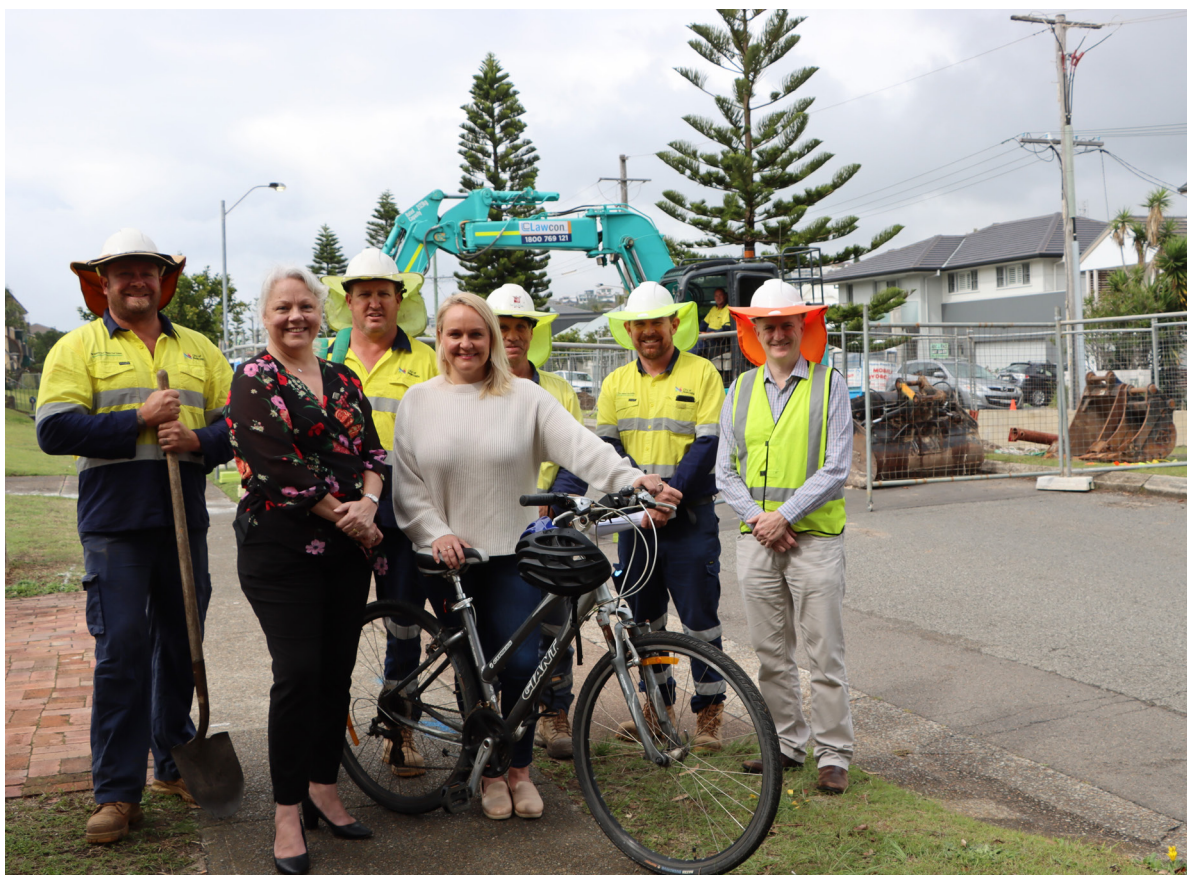
Councillor Carol Duncan and Newcastle Lord Mayor Nuatali Nelmes celebrate the start of the cycleway's construction with workers at the site
