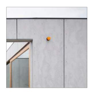
WALL CLADDING - 1 (FC.01) Fibre cement sheet
