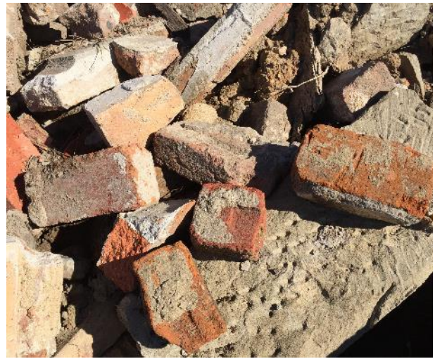
Figure 17 Hand cut stone, sandstock and dry pressed bricks with cement and lime mortar
