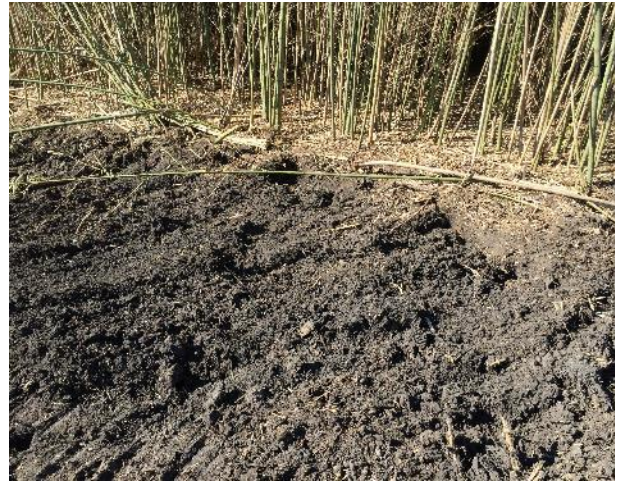
Figure 21 Removal of the bamboo and a maximum of 30cm of top soil
