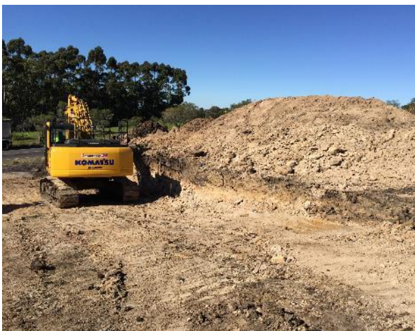
Figure 24 View east driveway to Murray Dwyer Circuit
