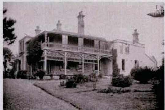
4. View of southern side of the Gregson House. Note what appears to be a Bunya Pine in the far left of the photograph. (Source: http://uonccmayfield.files.wordpress.com ).
