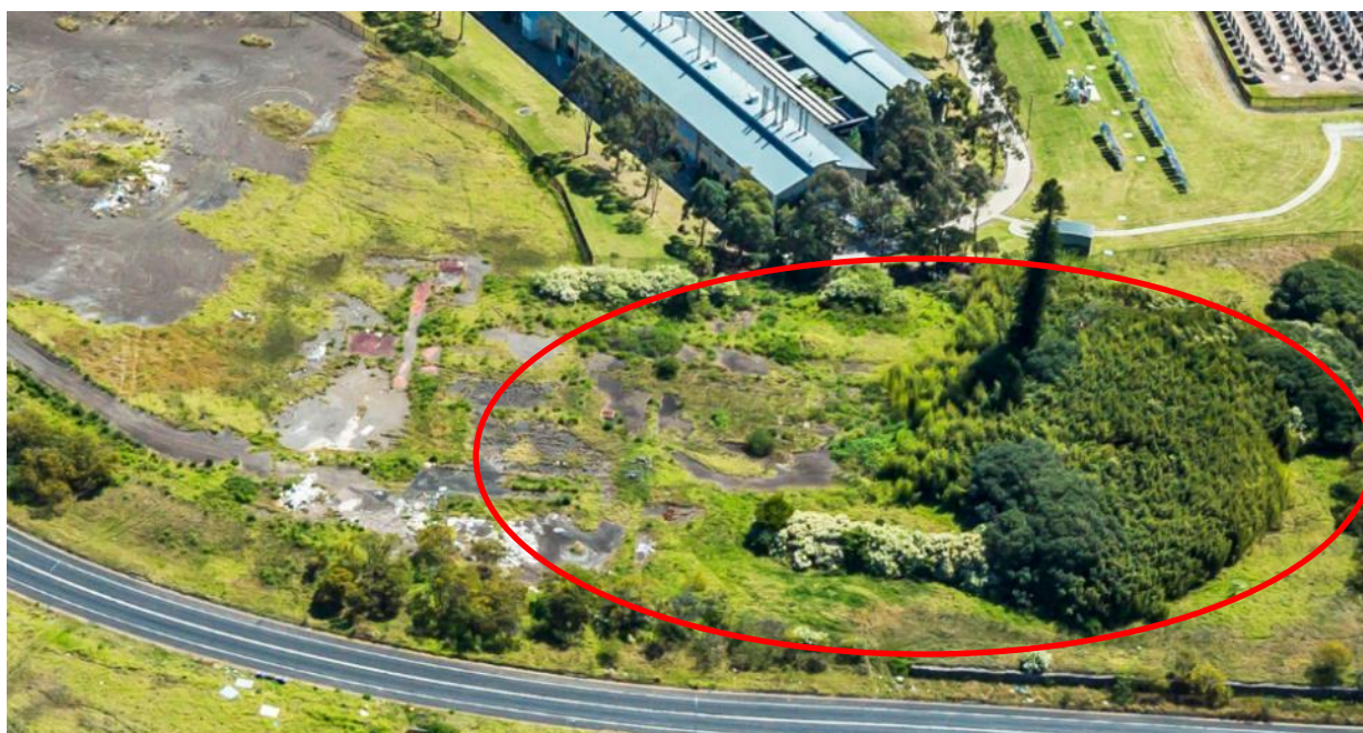
Figure 6 Location of the area of works showing the garden and remains of the orphanage in the ground (Colliers)
