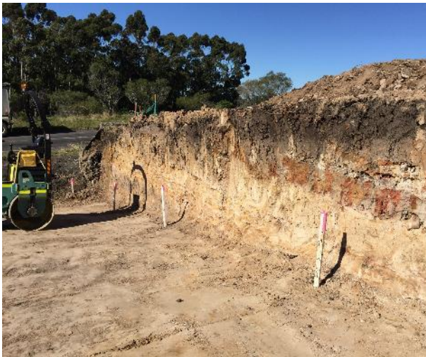
Figure 22 Excavation through topsoil and bedrock for the access driveway to Murray Dwyer Circuit on the eastern boundary
