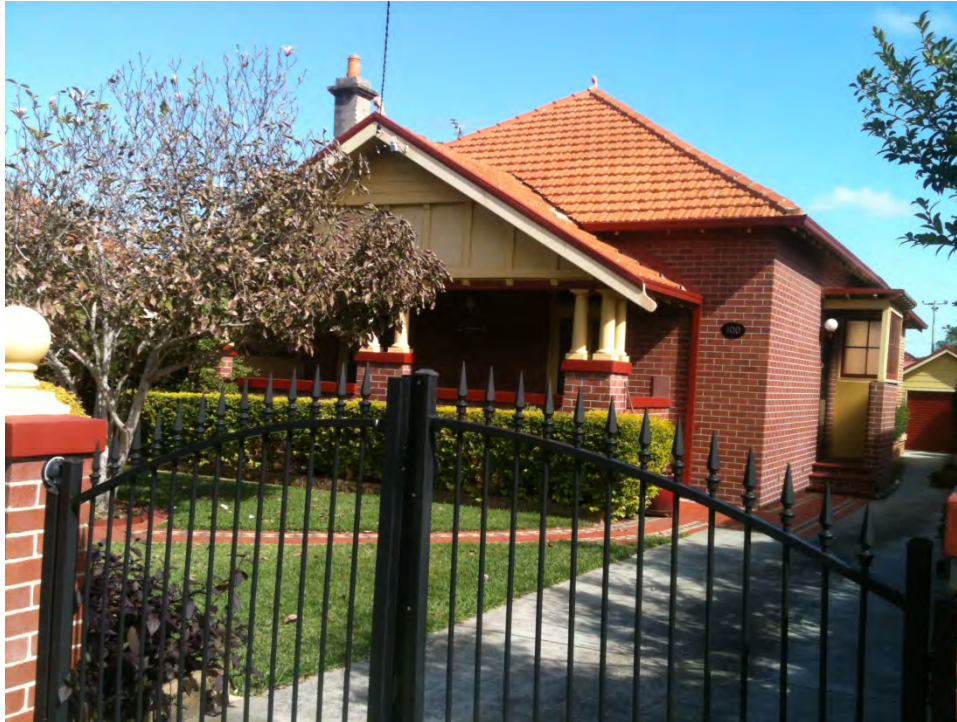
Figure 2.6 – A bungalow on Corlette Street. The dwelling contributes in a positive manner to the streetscape
