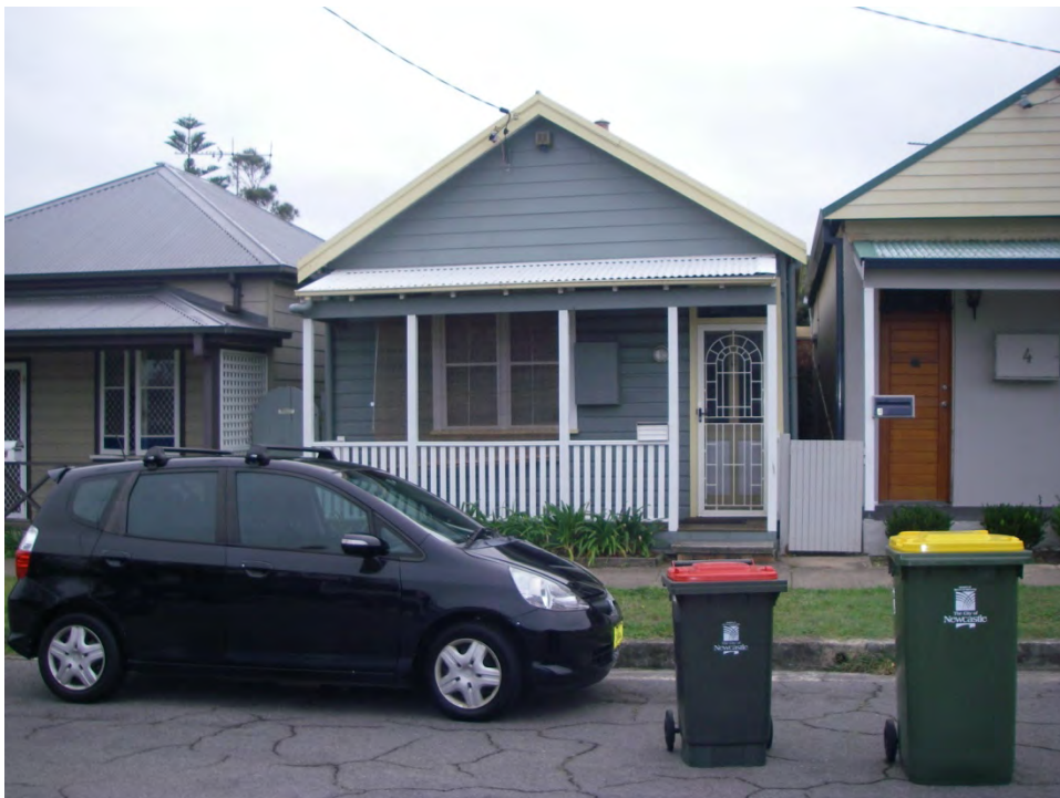
Figure 2.5 – A group of workers' cottages on Young Street
