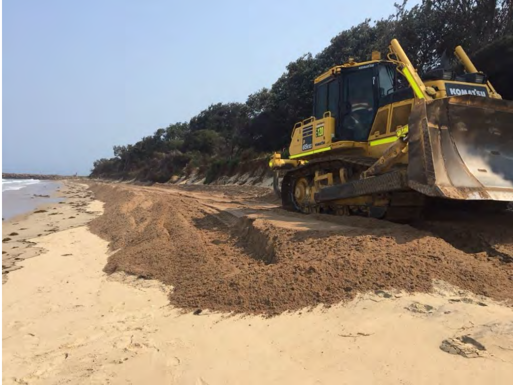
Figure 3: December 2019 nourishment activity in progress (date: 10/12/19)
