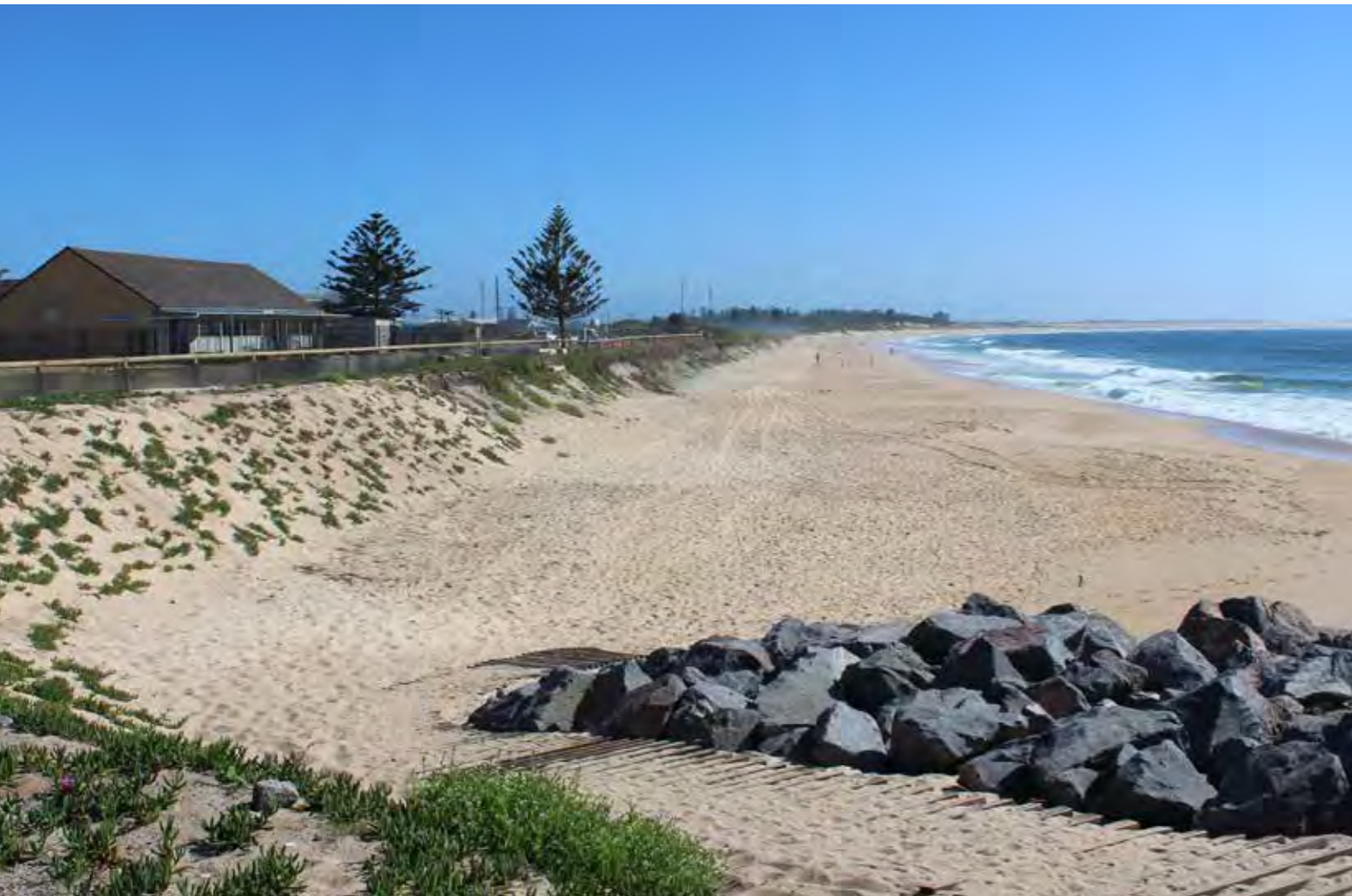
Figure 6. Northern section of Stockton Beach from northern end of Mitchell Street seawall. Former North Stockton Surf Life Saving Club building on back dune area now removed. (Photograph: MManning, CN, 4/1/19).
