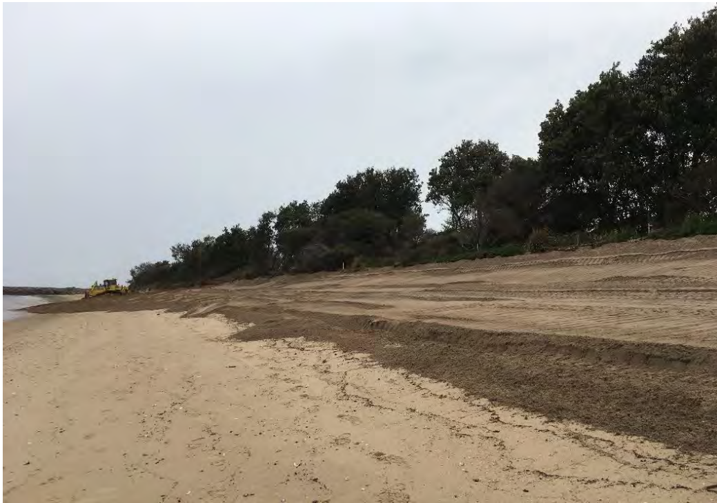
Figure 4: December 2019 nourishment activity upon completion (date: 12/12/19)
