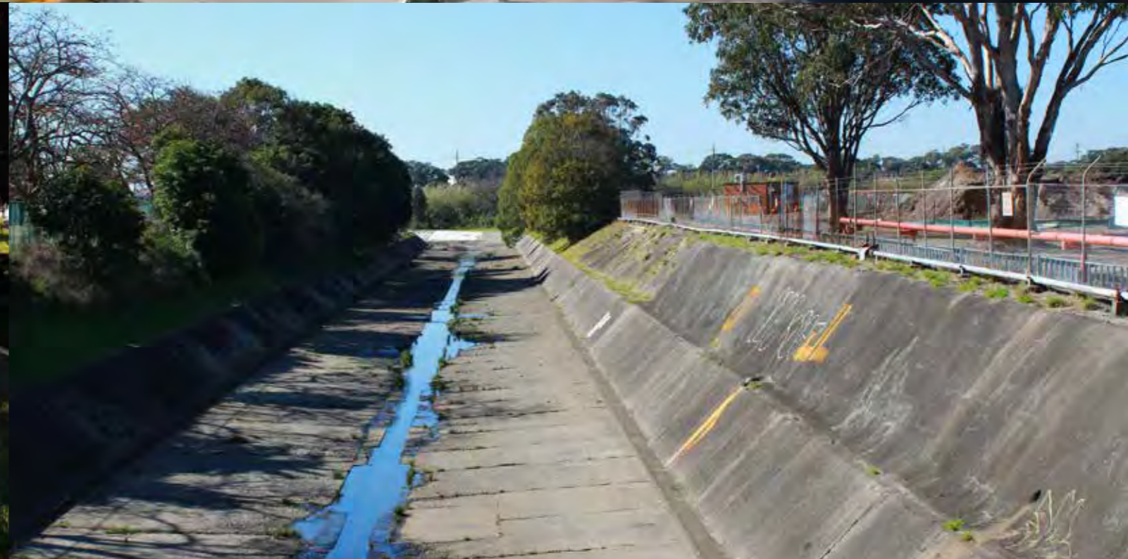
Figure 41. Styx Creek (stormwater channel) looking east from Chatham Road, Hamilton North. Former gasworks remediation site is to right of photograph. (Photograph: MManning, CN, 21/7/19).
