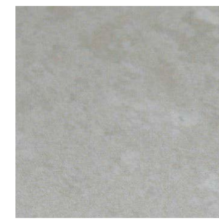
Unpainted Fibre cement sheeting to exterior and interior walls of addition
