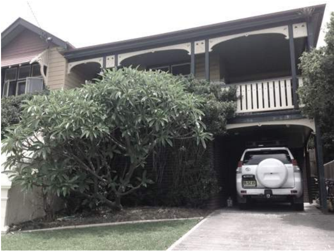
5. Front façade, north east corner
