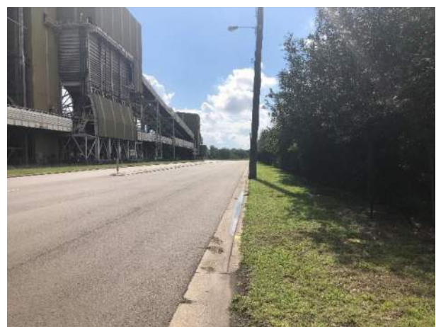
Figure 3.3.4b: Visibility to North from Driveway
