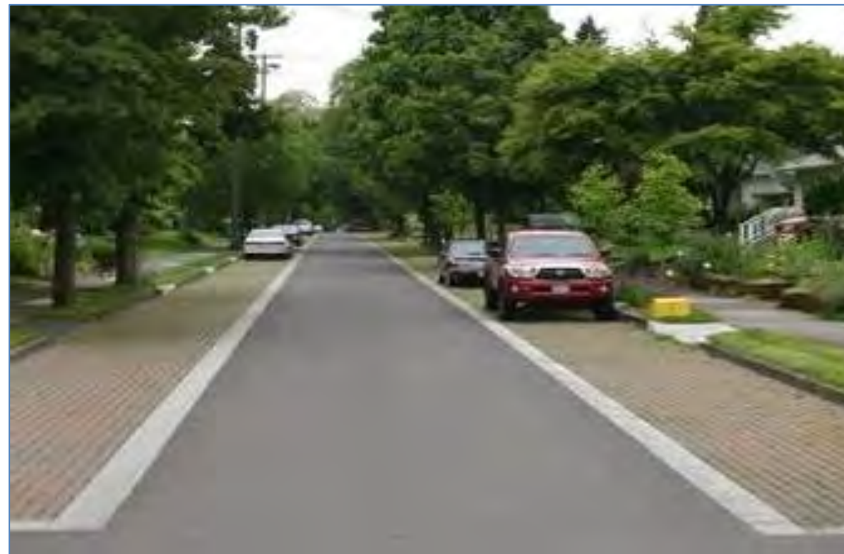
Figure 35 -An example of pervious paving applied to define on-street car-parking areas and facilitate stormwater management.
