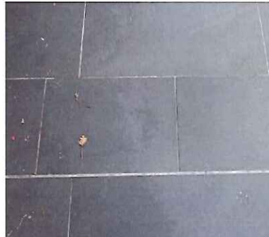
BLUESTONE PAVING TO BE DRAWN INTO PLAZA FROM HUNTER STREET PROVIDES PEDESTRIAN LINKAGE
