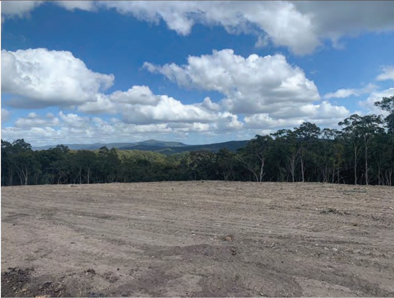
Photo taken from future Walker Crescent, Fletcher looking directly west over the site.
