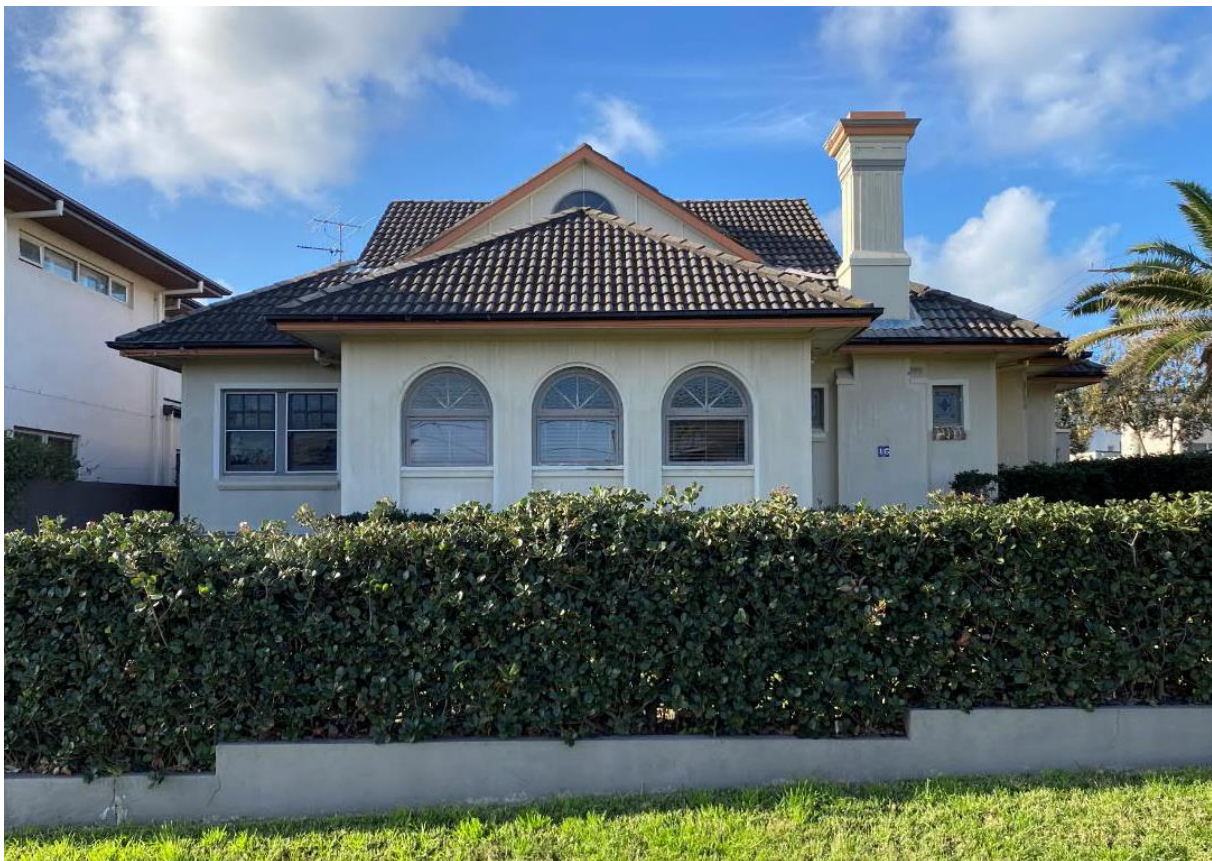
Figure 12: South Elevation from Parkway Avenue showing the distinctive arched windows & half round roof tiles (Source: EJE)
