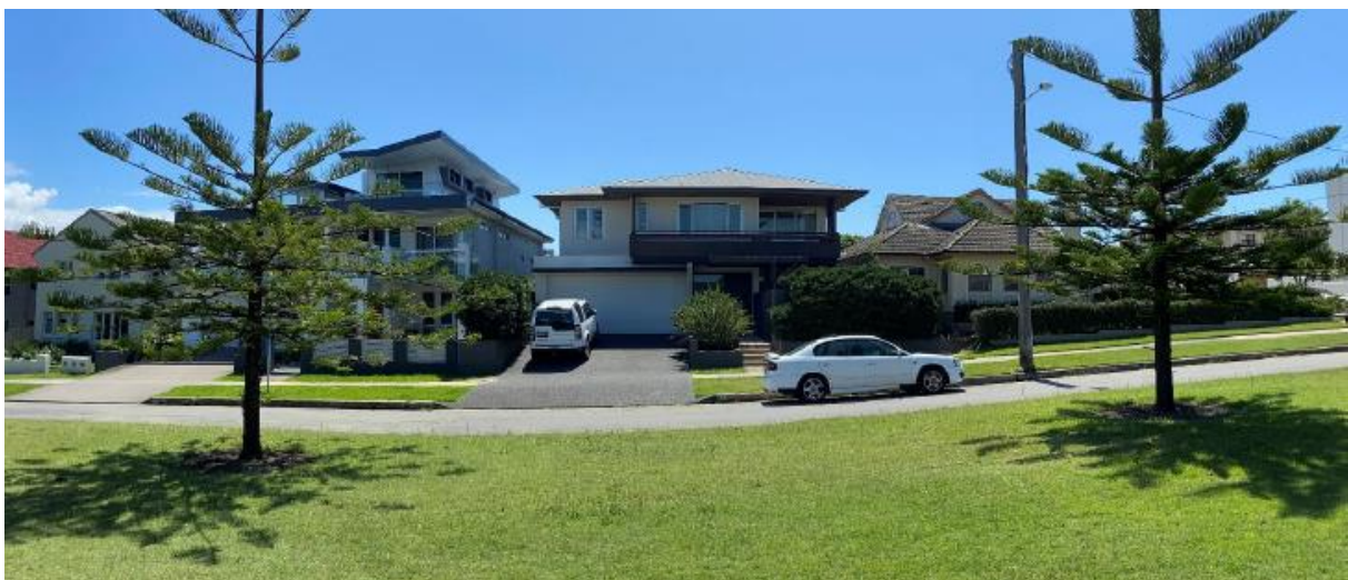
Figure 10: Streetscape photo of No's 16, 18 and 20 Parkway Avenue (Source EJE Architecture)
