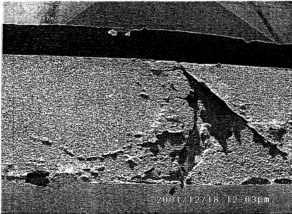
Photograph 12180109 Erosion of patch in render, with paint failure
