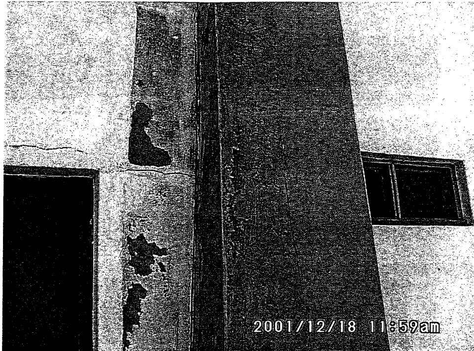
Photograph 12180092 Failure of paint over recent column repair (sea-side)
