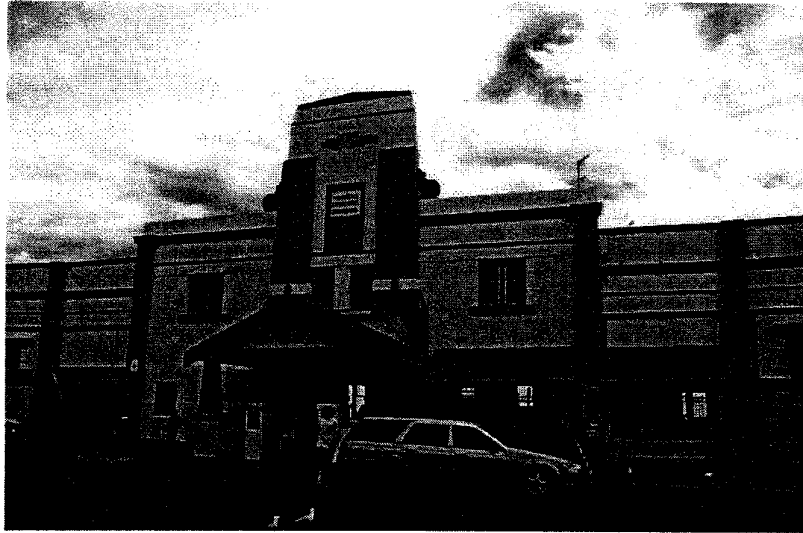
Figure 3.3 The west elevation of the Baths Pavilion. source: Suters Architects
