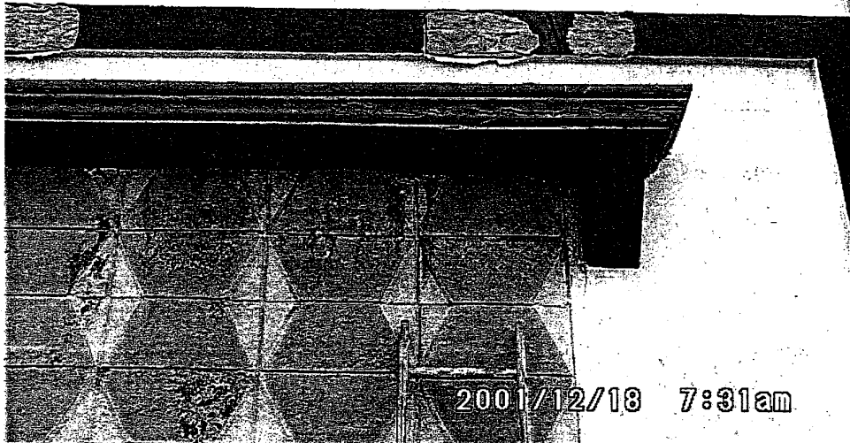
Photograph 12180012 Sun-hood over patterned in-fill, believed to be a filled in opening in the facade
