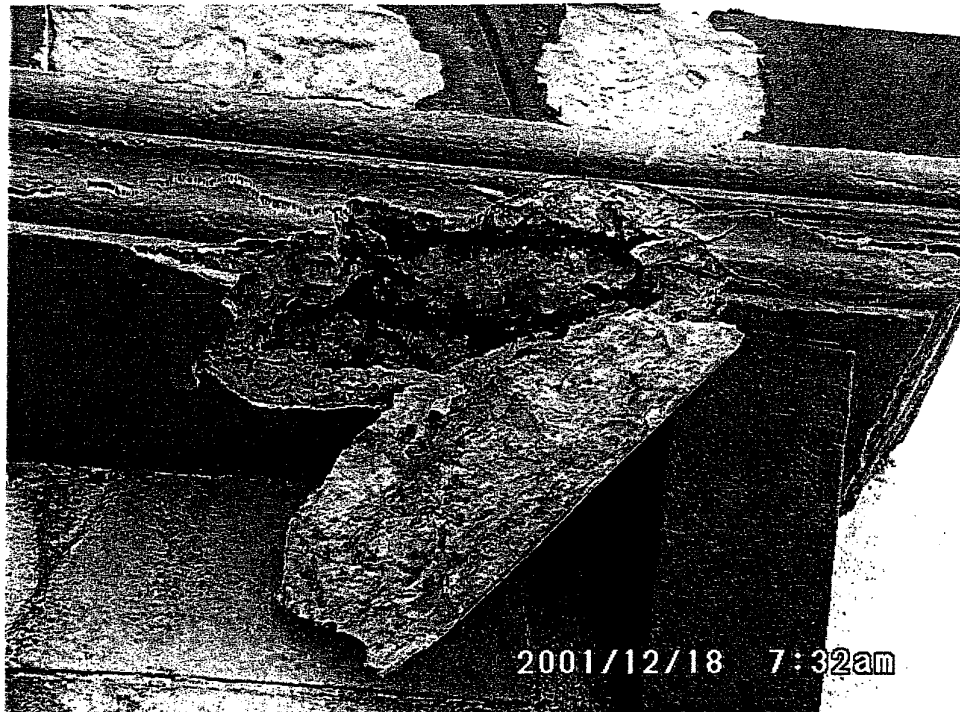
Photograph 12180013 Delamination of cover concrete at drumminess
