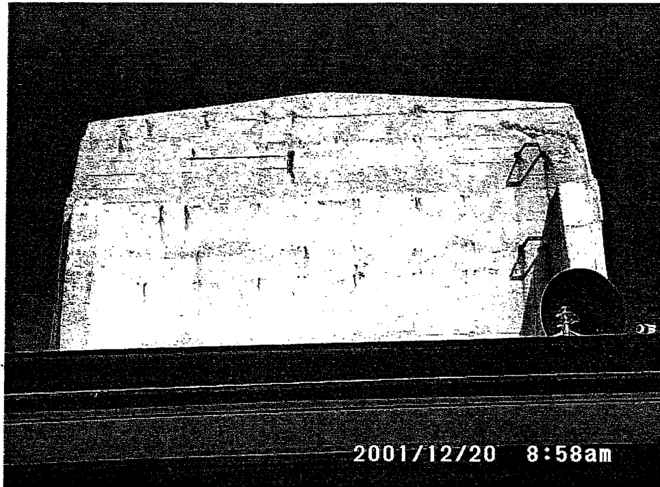
Photograph 12200001 Rust spots and old spalls in rear of facade
