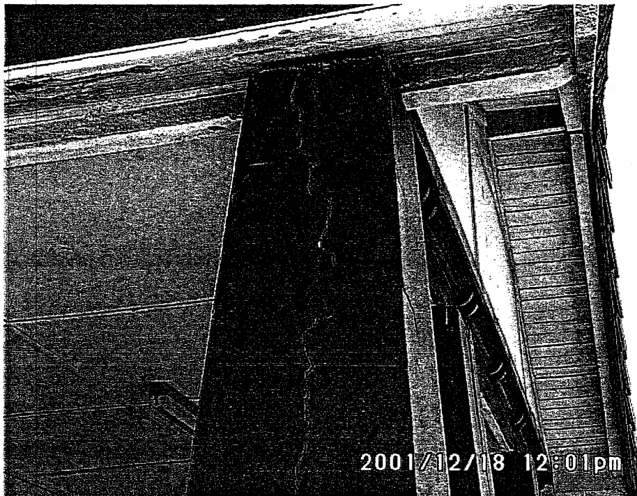
Photograph 12180104 Cracking in columns to main entrance porch
