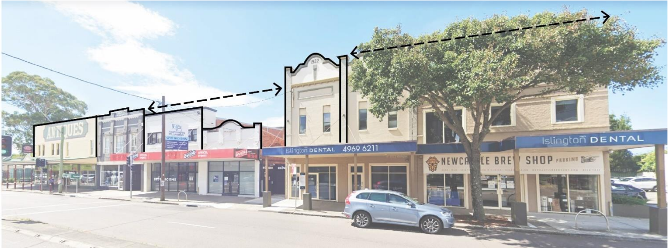
Figure 36: Existing parapets dominating the street edge
