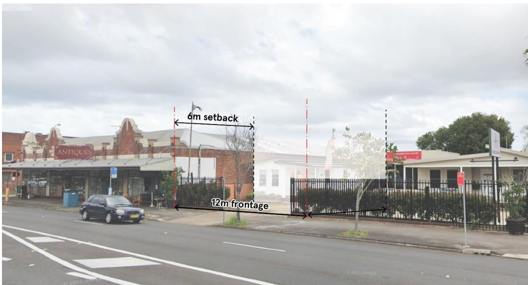
Figure 26: Development adjacent to the Coliseum
