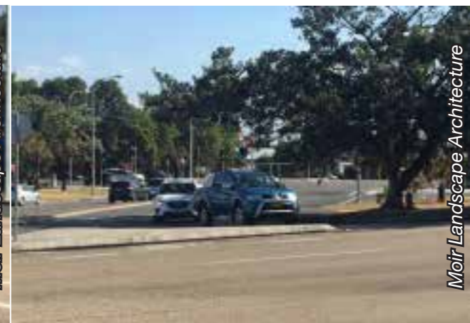
Selma Street slip lane onto Hunter Street
