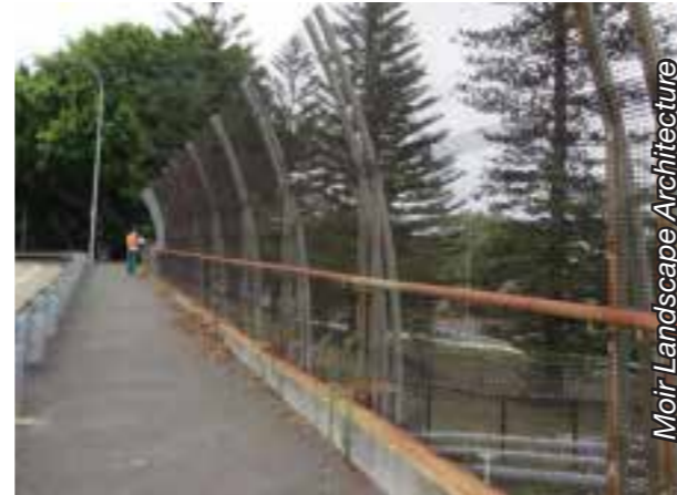
Rail bridge overpass, Hunter Street
