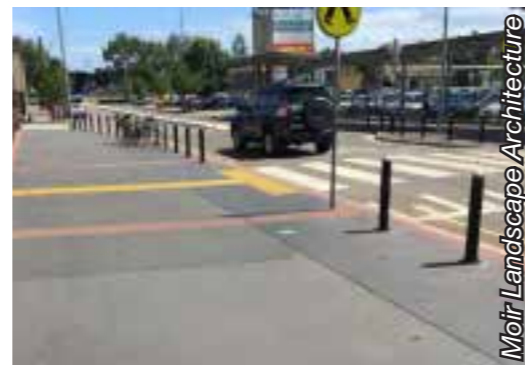
Marketown pedestrian crossing, Steel Street
