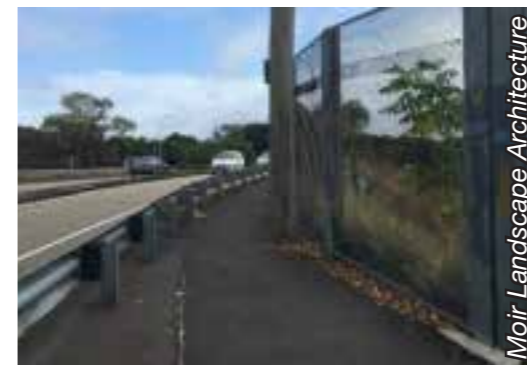
Railway bridge, Hunter Street
