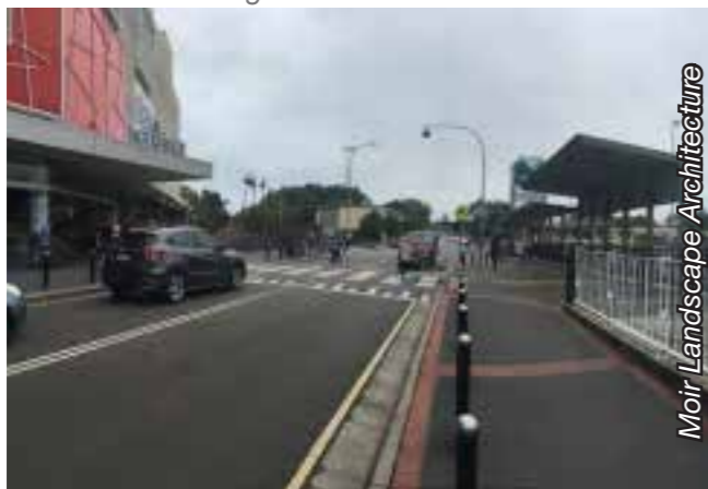
Pedestrian crossing at Cottage Creek
