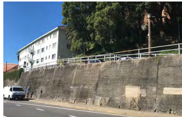
Image: The City's Smart City Strategy provides a roadmap for deploying new technologies across the NAPA that can nurture artists and activate the built environment. Sites such as the 'King Street Wall', at the corner of King and Darby Streets, can be transformed into a digital canvas using interactive technologies. Source: Author's collection.
