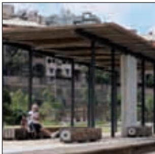
Shade structure, Pyrmont Park
