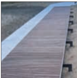
Timber walkway, Ballast Point
