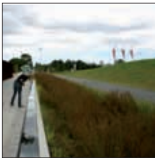
Swale, Armory Wharf
