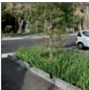
Parking bay swale and tree planting
