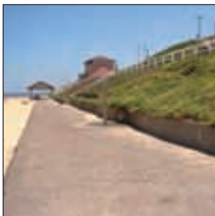
Sloped bank, retaining wall and promenade
