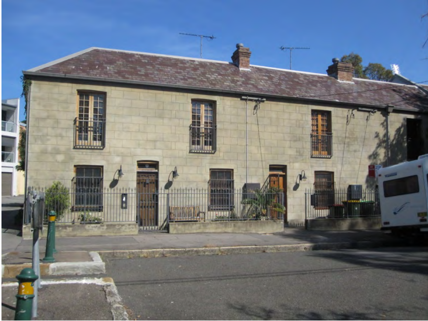
Figure 2.3 - Georgian style attached terraces on Queen Street
