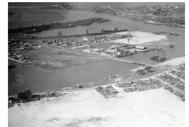
Figure 4 A view of Carrington showing land reclamation works, circa 1930. (Source: Milton Kent collection)
