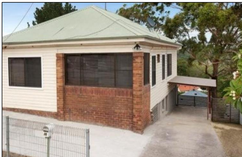
Figure 2: Existing dwelling showing the carport on the northern boundary
