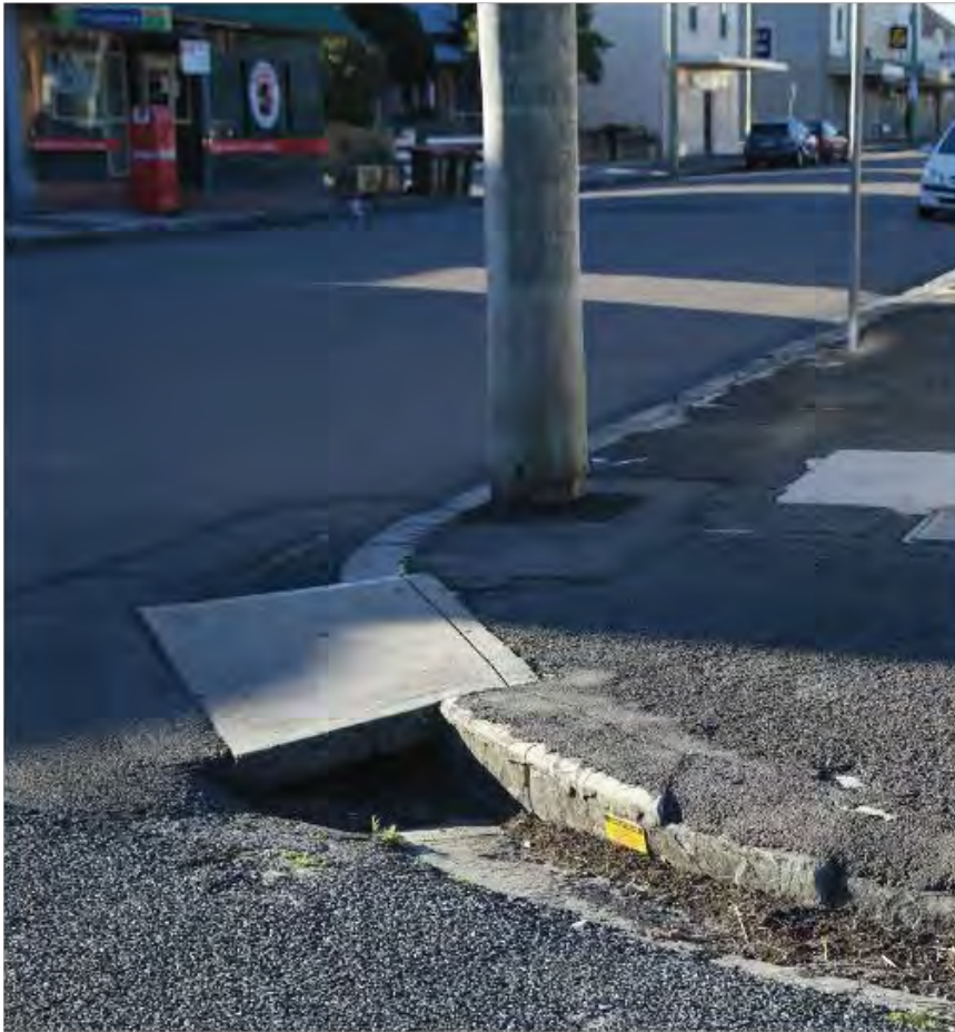
Storm-water flows below existing kerb ramps
