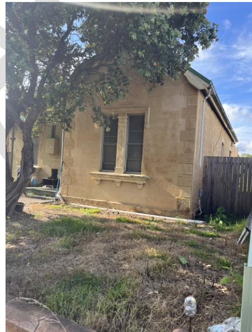
Figure 11. 14 Sunderland Street Mayfield front gabled roof and decorative mouldings around the windows
