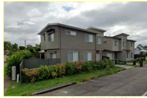
41 WILLIAMSON & 18 JOHN STREET TIGHES HILL
