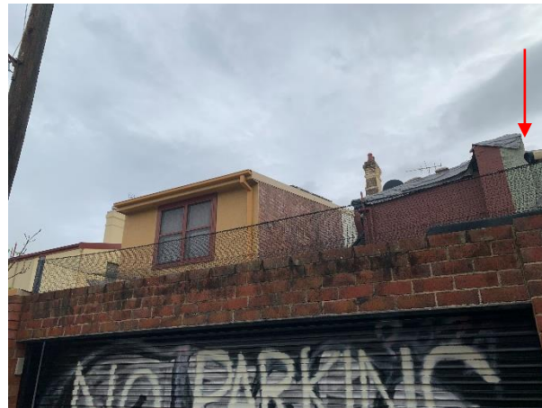
Figure 4 The adjoining neighbour to the west (subject property indicated).
