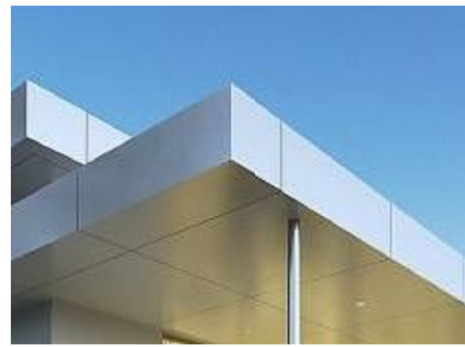
PREFINISHED METAL SHEET FASCIA CLADDING. LIGHT COLOUR
