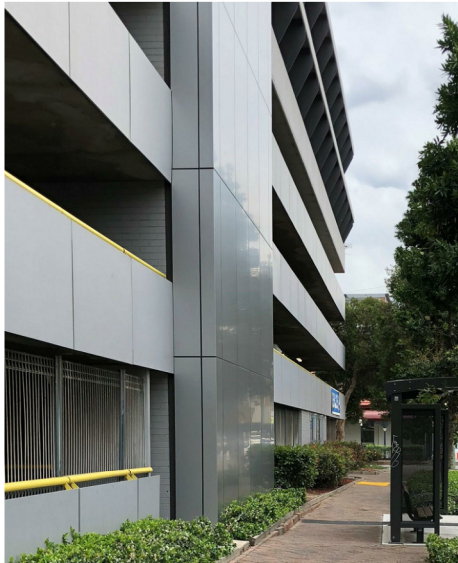
PAINTED SHEET SILL/SPANDREL - TO MATCH EXISTING LEVEL 5 & 6
