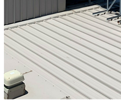
METAL DECK ROOF SHEETING. LIGHT COLOUR
