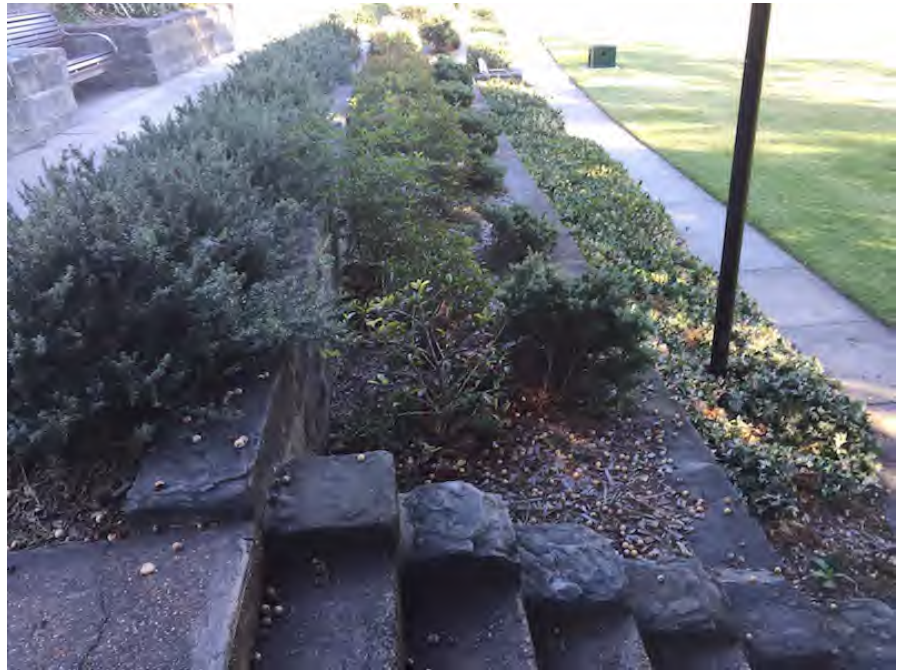
Concrete stairs from Laman Street at eastern end of sandstone Terrace
