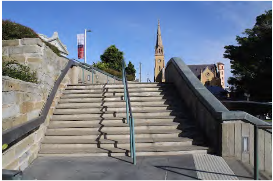
Balustrade and stairs in area of fountain
