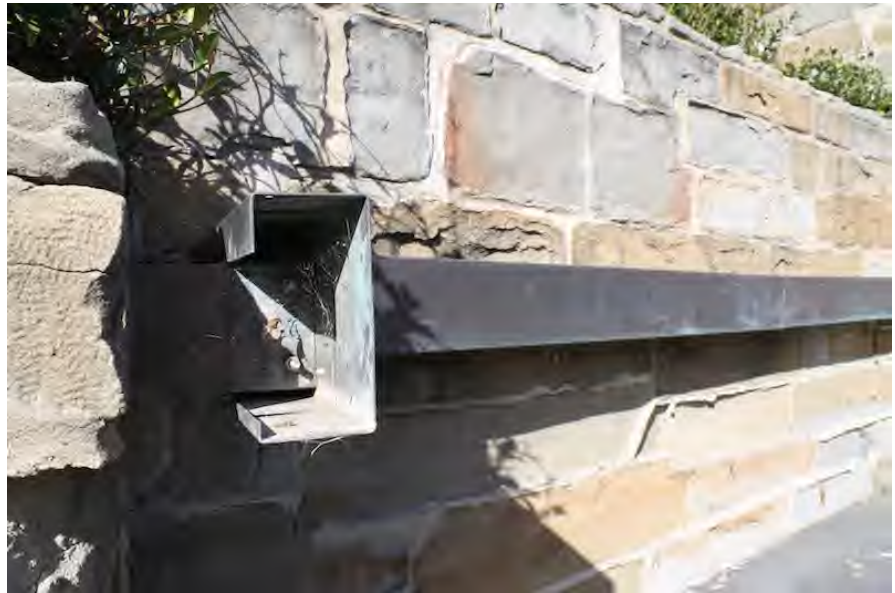
Balustrade in area of fountain
