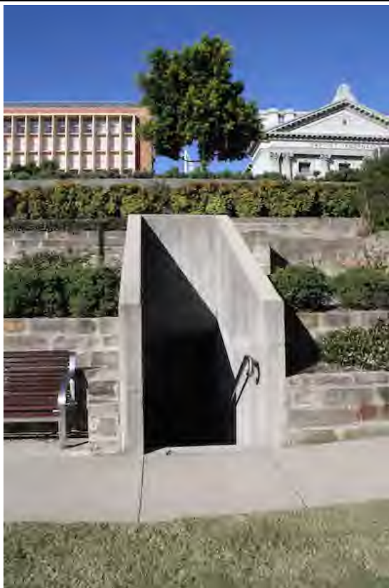
Access to service area to west of the fountain.
