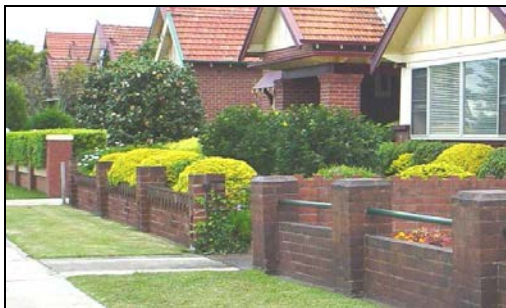
A typical palette of materials including terracotta roof tiles, and tuckpointed brickwork with matching fences is evident in this group of California bungalows.
