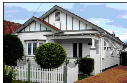
A good example of a weatherboard bungalow with a double gable and matching picket fence
