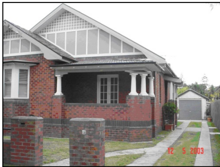
Typical double gable roof on a California Bungalow
