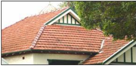
A typical roof treatment- unglazed Marseilles pattern terracotta roof tiles and half timbering to the gable ends.
