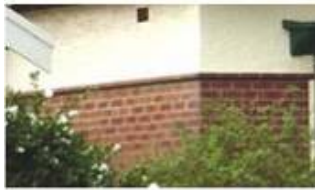
Some bungalows feature polychromatic exterior treatments such as tuckpointed face brick and pebbledash on the upper portion of the wall surface.
